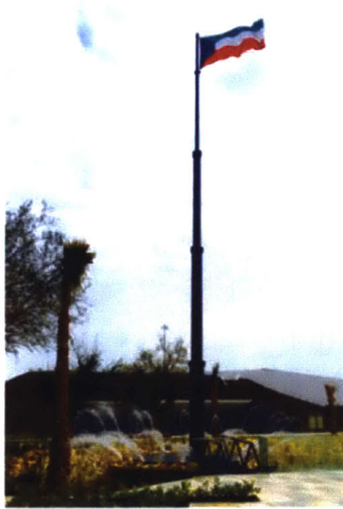
Telescopic Flagpole, Designed to be raised during events.
