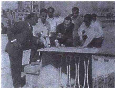
On-site Design and Construction efforts by Shiber for the Municipality Garden
