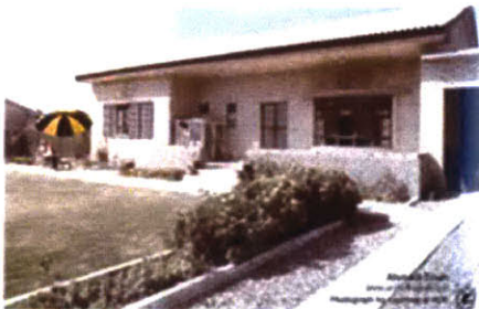
Typical Ahmadi Home housing British and American Workers
