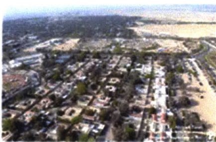
General View of Ahmadi Landscaping, 2010
