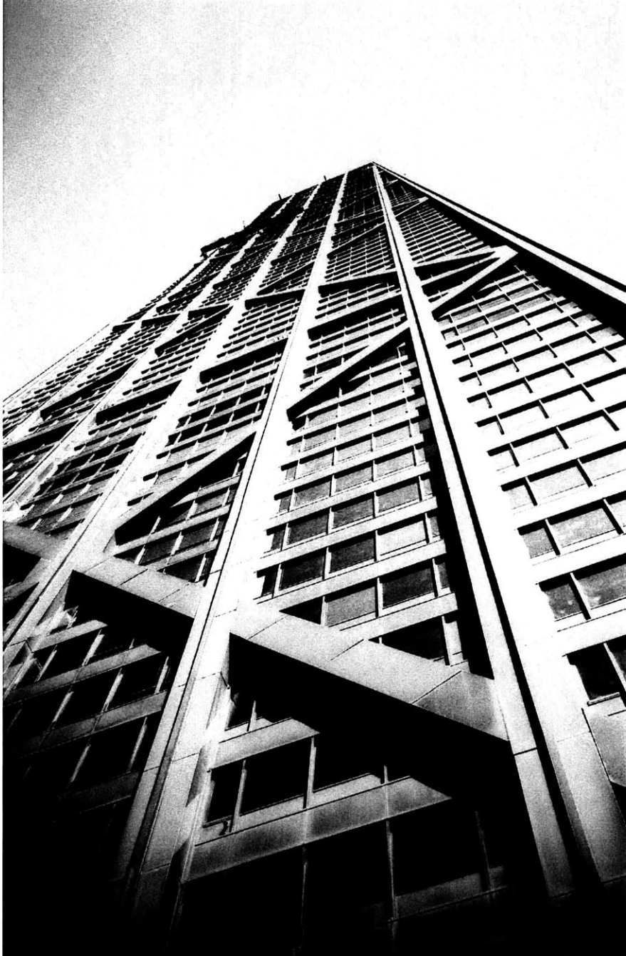
Figure 06.13 John Hancock Center, Chicago, Illinois
