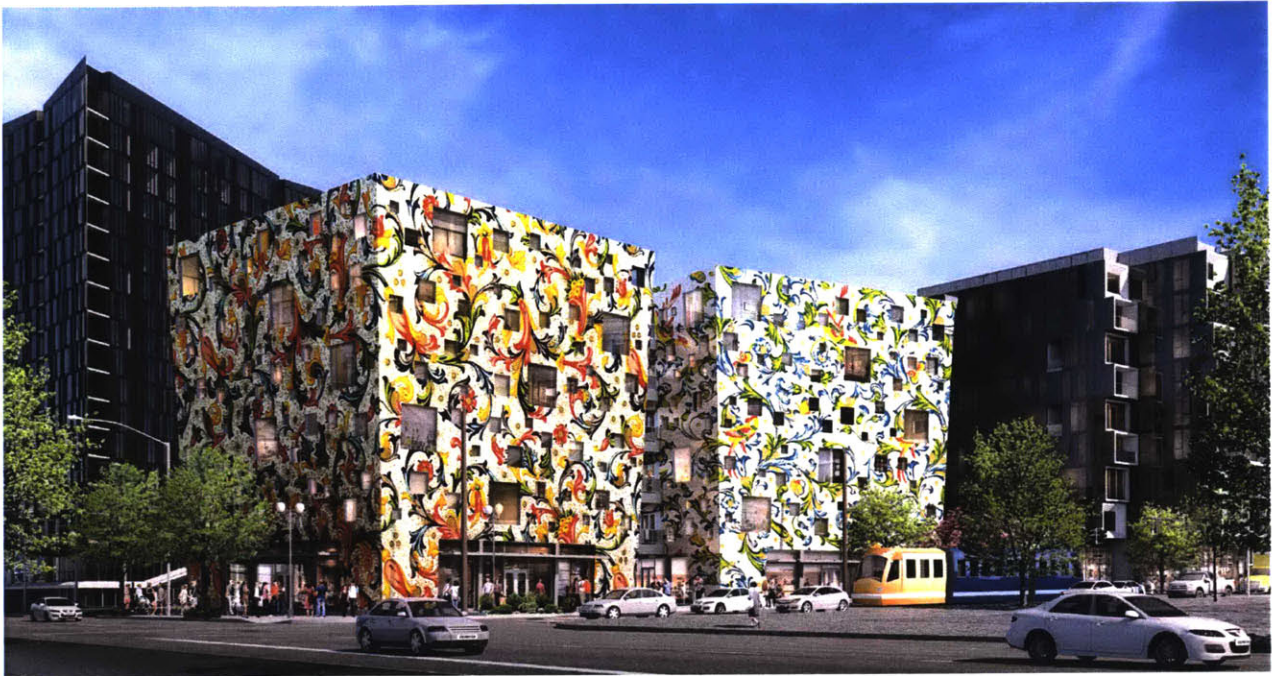
Figure 04.1 Guerrilla Development's "Fair Haired Dumbbell", Portland, Oregon, 56,000 square foot speculative office building
