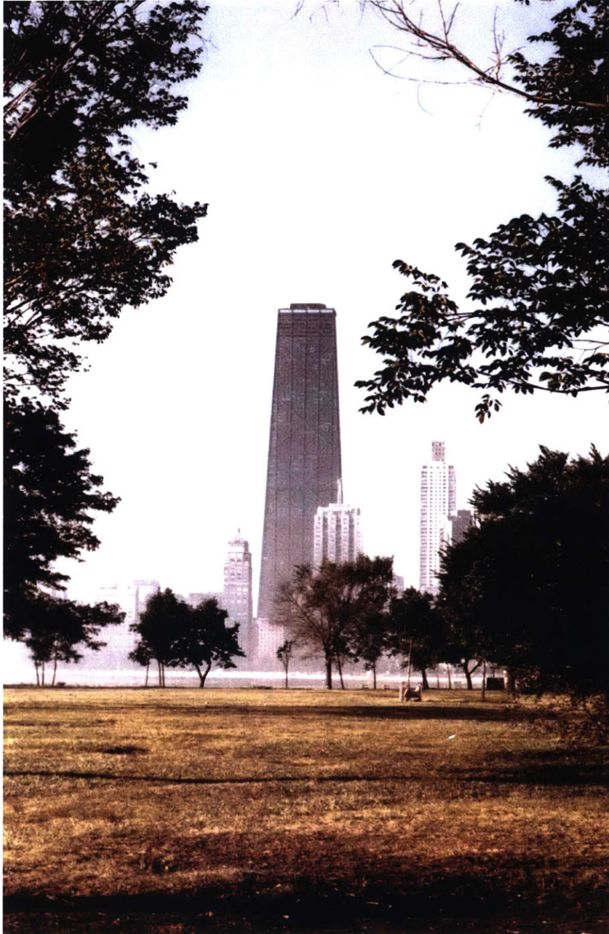
Figure 03.3 John Hancock Center, Chicago, Illinois
