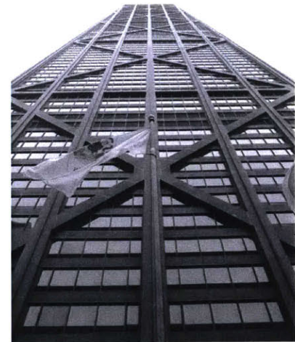
Figure 02.2 John Hancock Center Exterior, Chicago, Illinois
