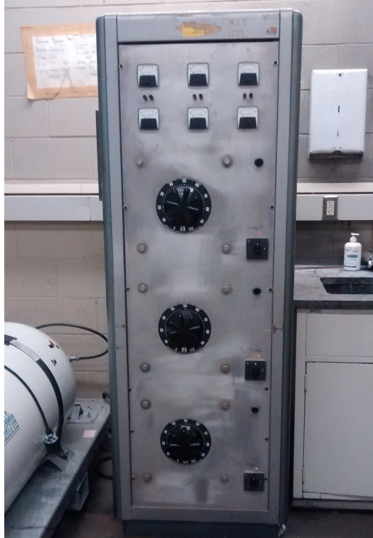
Figure B-16: 208V 3-phase VARIAC cabinet used to control the heating tapes
