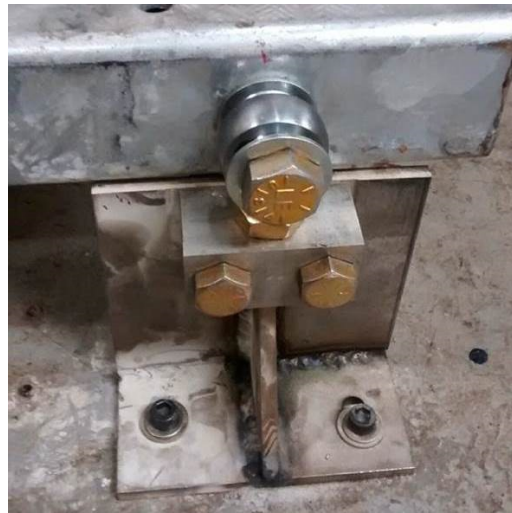
(b) Spherical bearing tank mount
