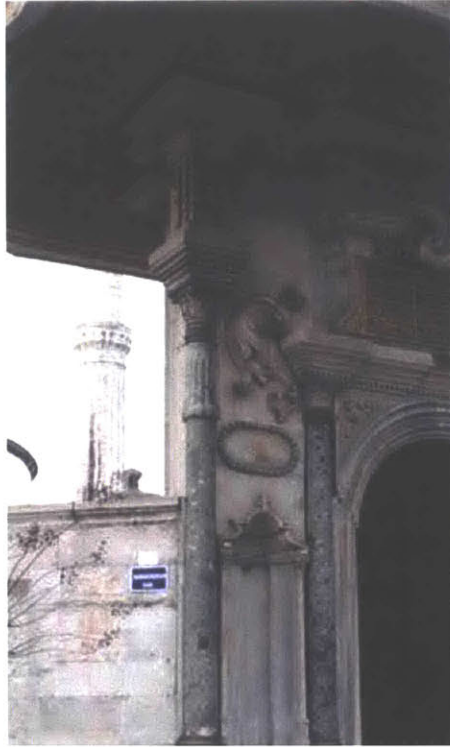
Fig. 4.13 Detail of the gate of the Hagia Sophia Public Kitchen (1743).
