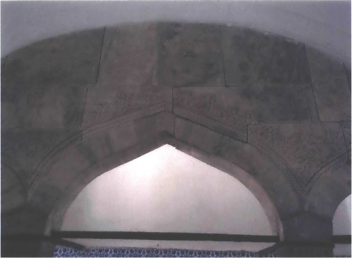
Fig. 2.13 Detail of the arcade in the Şehid Ali Paşa Library.
