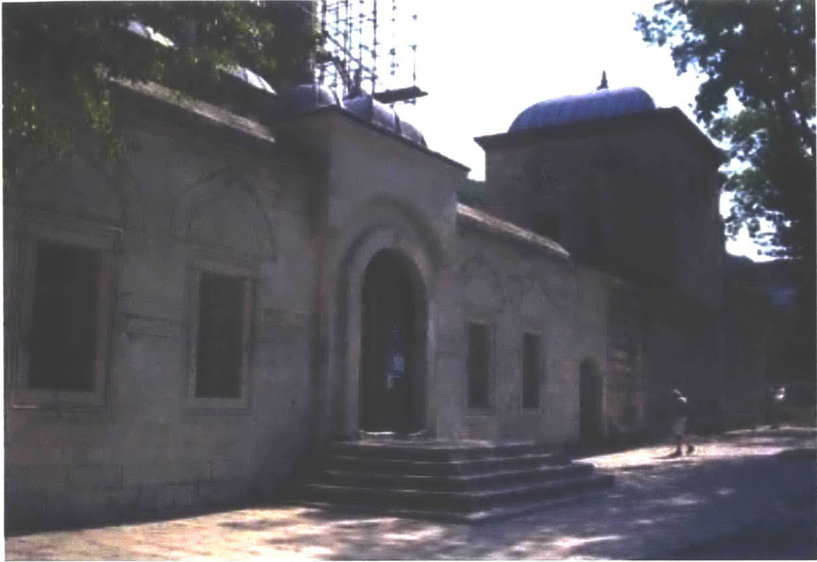
Fig. 1.25 Library in the Şerif Halil Paşa Complex in Shumen (1744).
