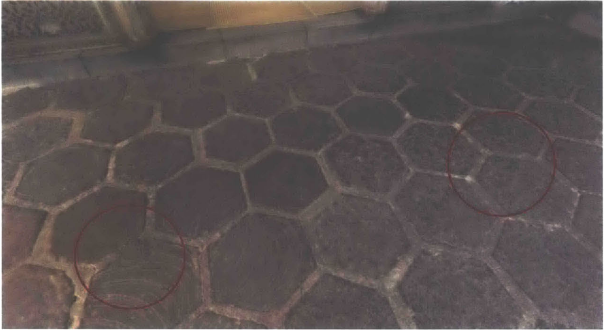
Fig. 2.26 Places of two feet of the original book depository in the Ahmed III Library (from the restoration report).
