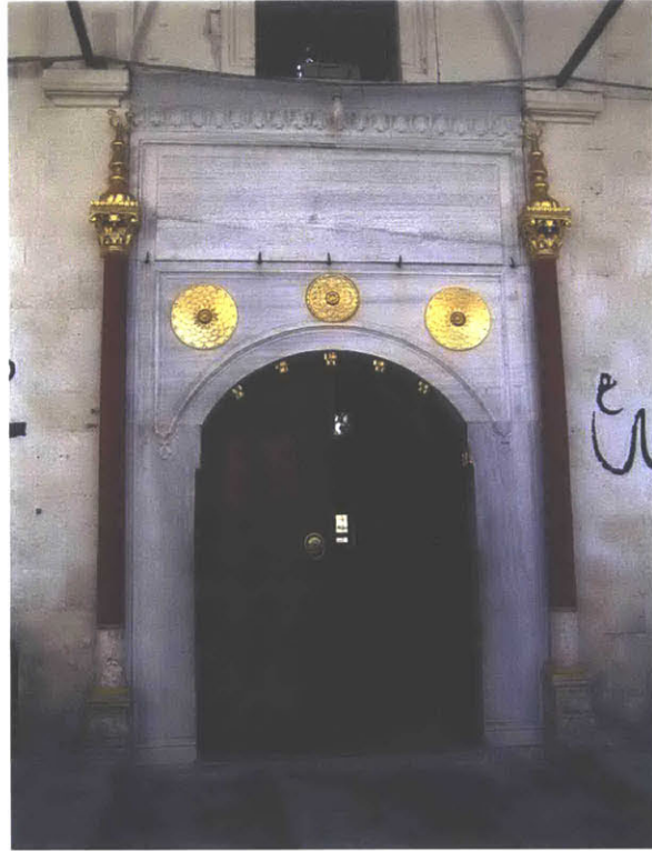
Fig. 1.23 Entrance to the Şerif Halil Paşa Mosque.
