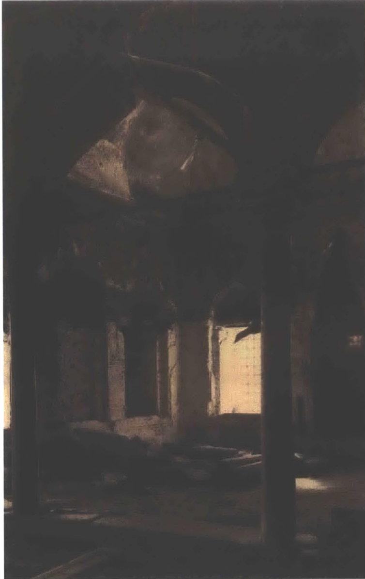
Fig. 2.8 Şehid Ali Paşa Library at Yerebatan, the main hall (Istanbul Committee of Historic Preservation Archive, file no: 0724).
