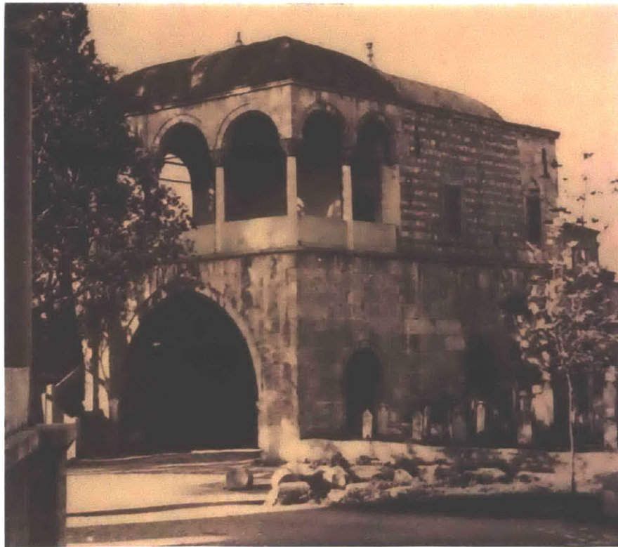
Fig. 1.34 Hekimoğlu Ali Paşa Library (from Goodwin, A History of Ottoman Architecture ).
