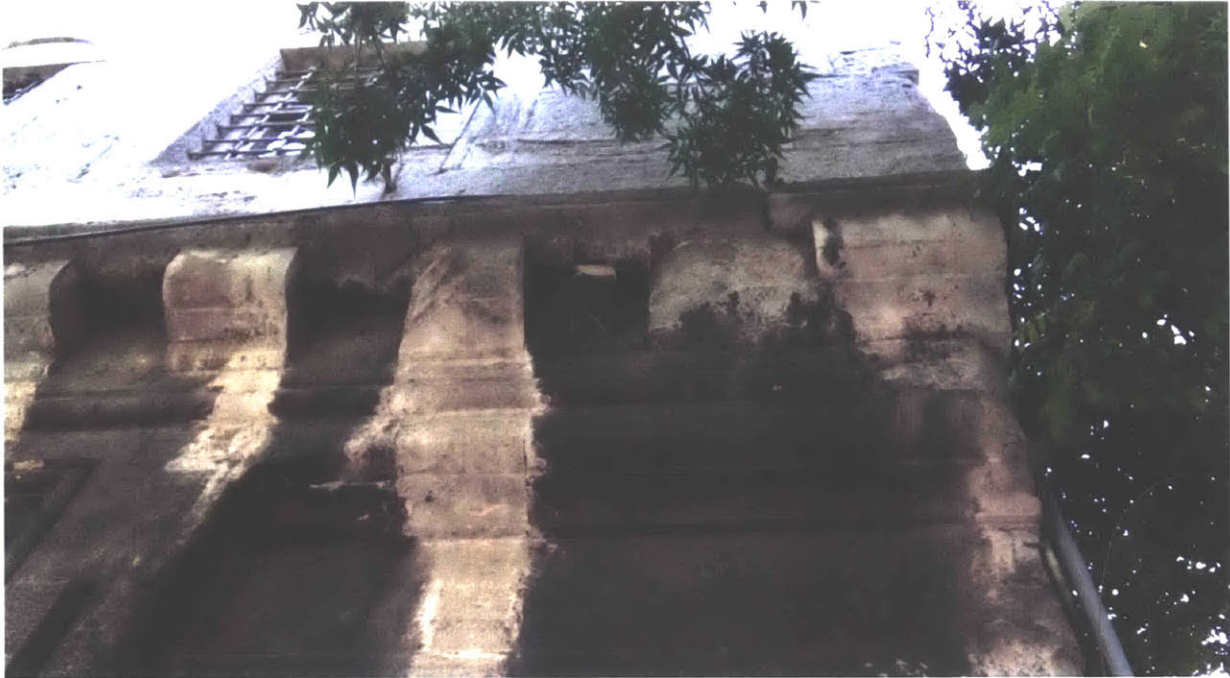
Fig. 1.31 Birdhouse on the façade of the Hekimoğlu Ali Paşa Library.
