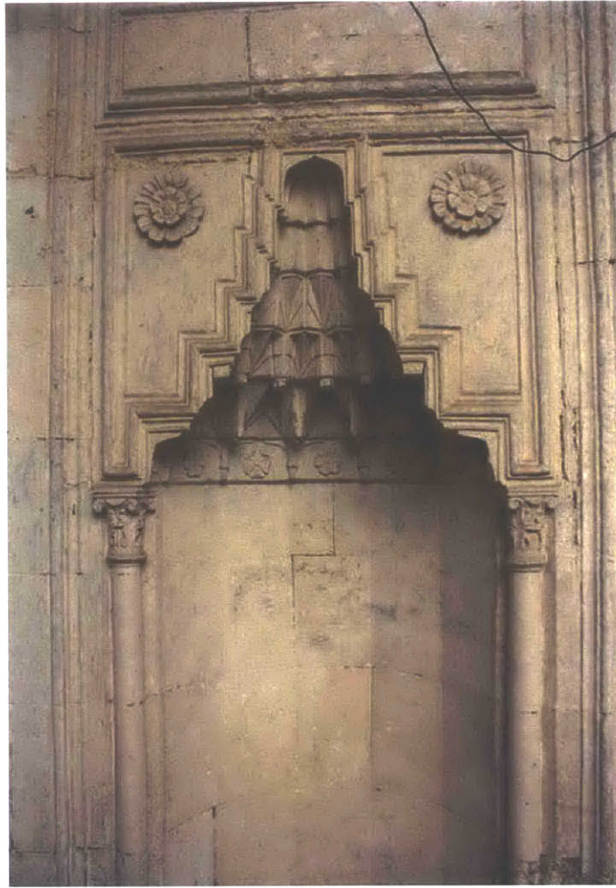
Fig. 1.22 Mihrab niche in portico of the Şerif Halil Paşa Mosque.
