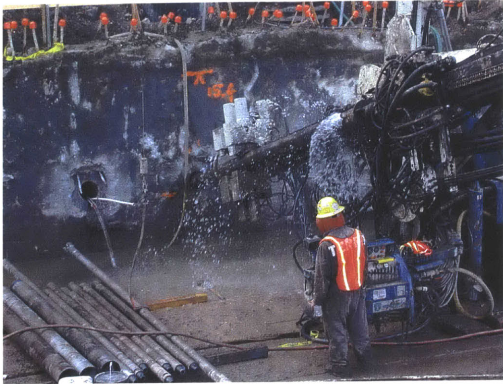
FIGURE C-20: Tieback drilling and exposed tieback sleeve, tendon, and grout tube.
