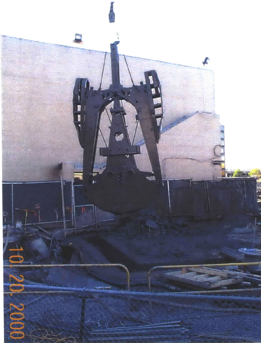
FIGURE C-18: Mechanical clamshell used to excavate wall panels.
