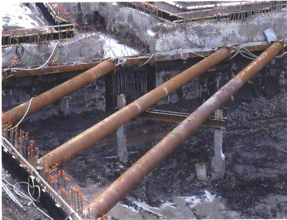
FIGURE C-23: Southeast corner bracing showing piles used to support the long braces.
