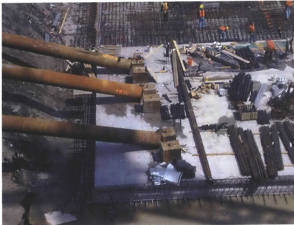
FIGURE C-27: Attachment of the rakers to the kicker blocks.
