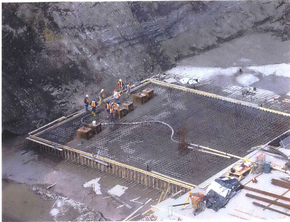
FIGURE C-26: Construction of a slab section with kicker blocks for the rakers.
