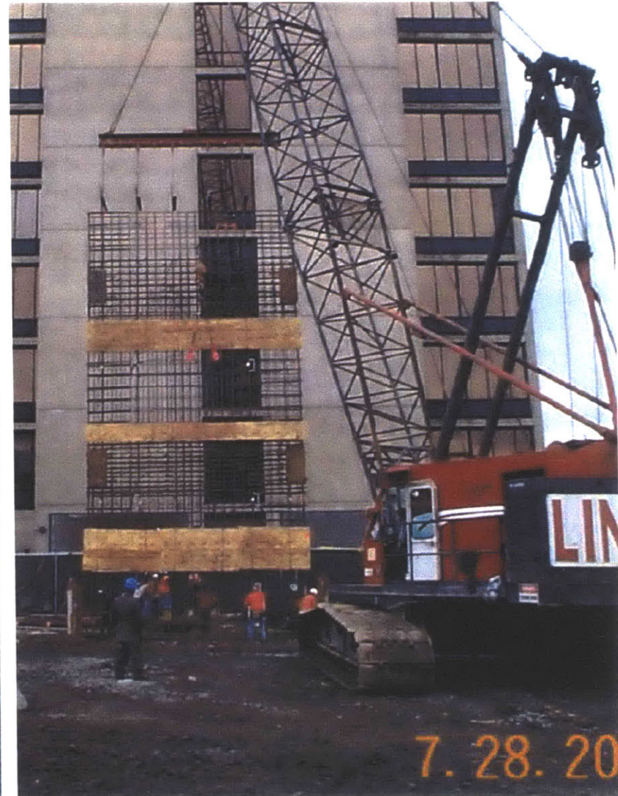
FIGURE C-19: Placement of reinforcement steel for a wall panel.
