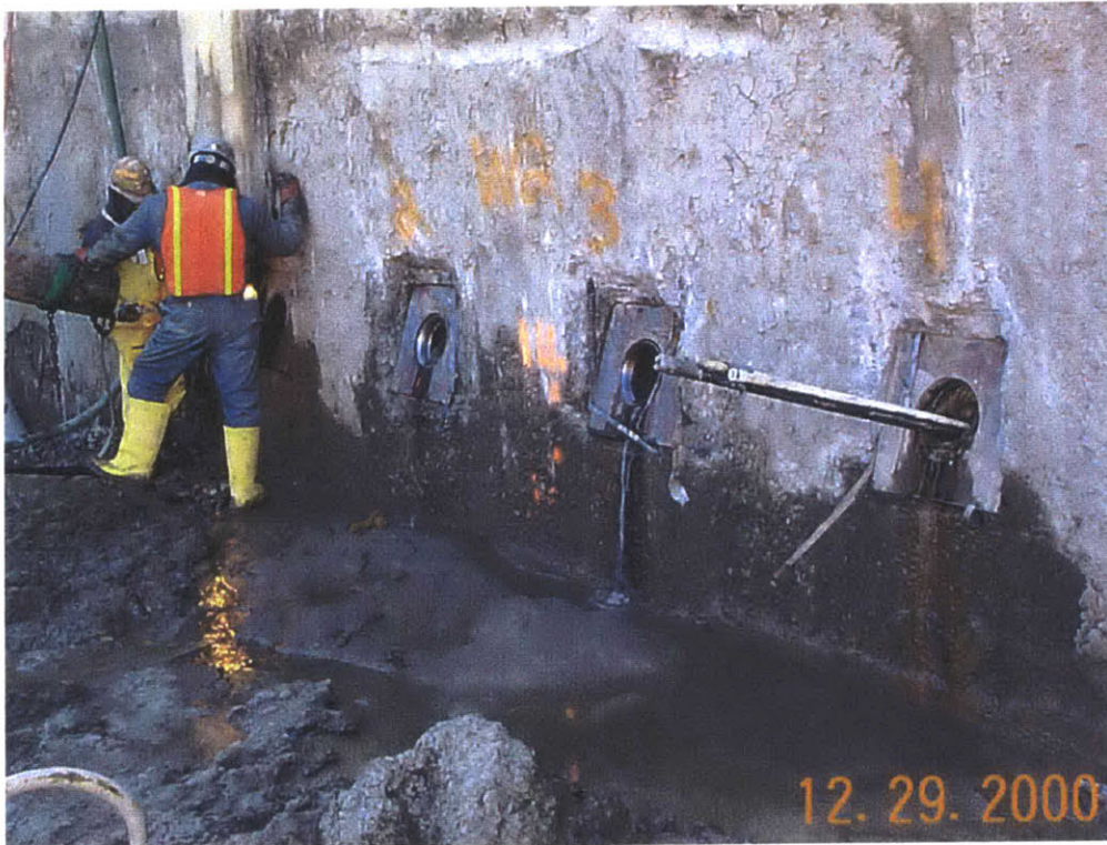
FIGURE C-21: Exposed Tieback Sleeves
