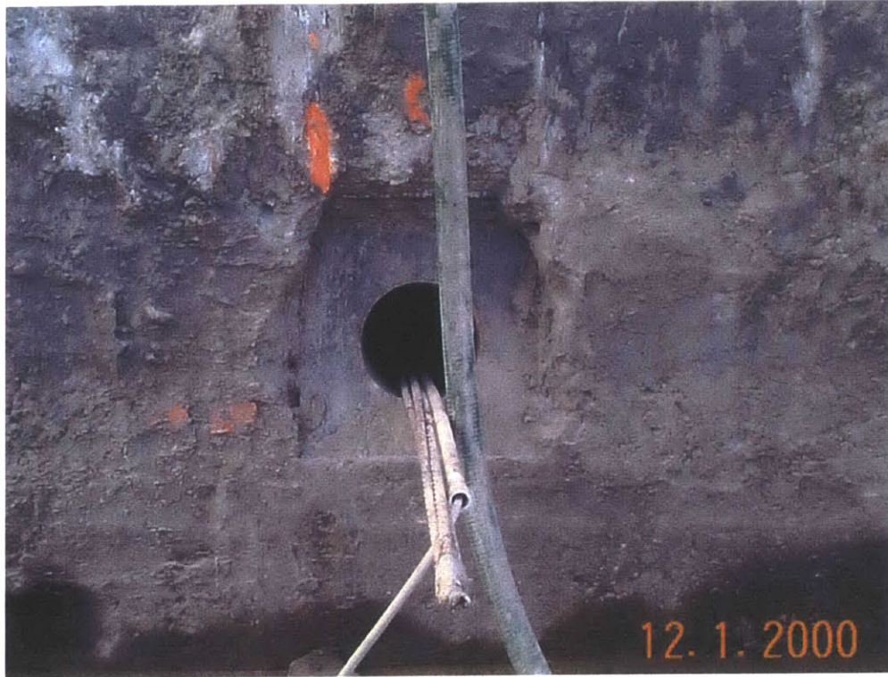
FIGURE C-22: Exposed tieback sleeve with tieback grouting in progress.
