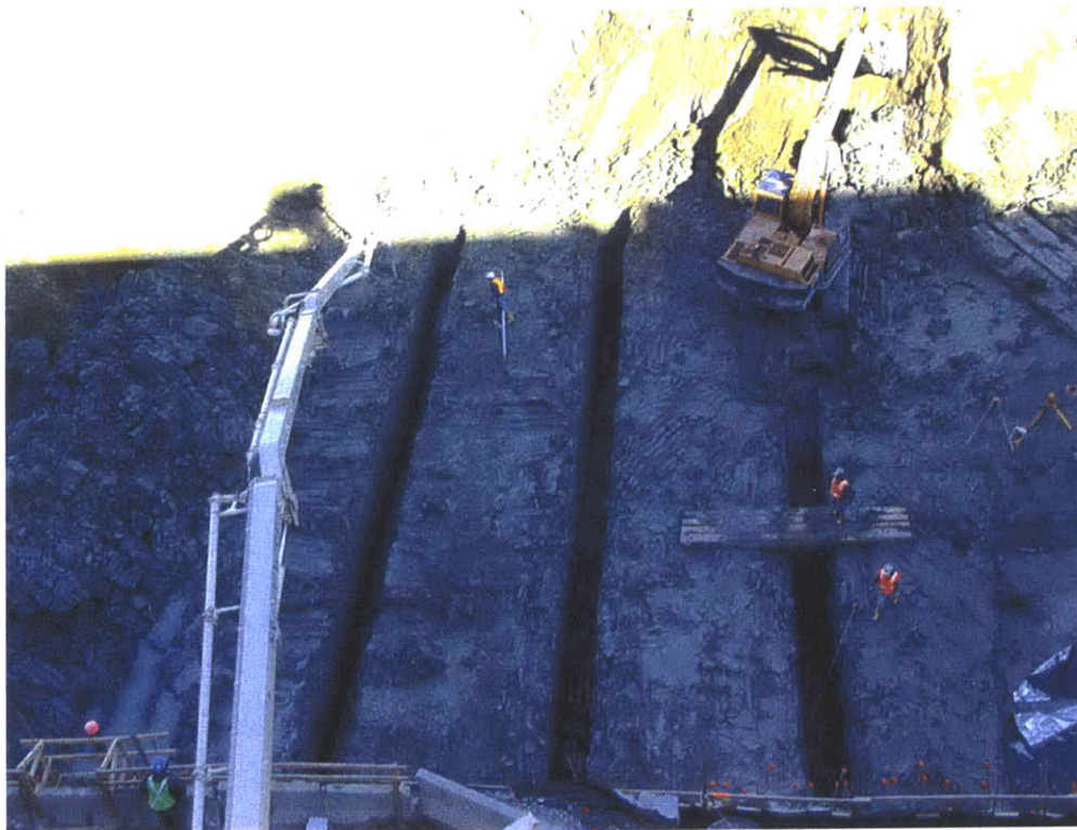
FIGURE C-28: Raker supports on the North wall with coverings to help protect struts from the heat of the sun.
