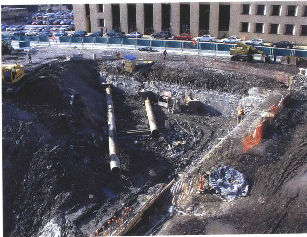
FIGURE C-25: Assembly of corner bracing in the Northeast corner.
