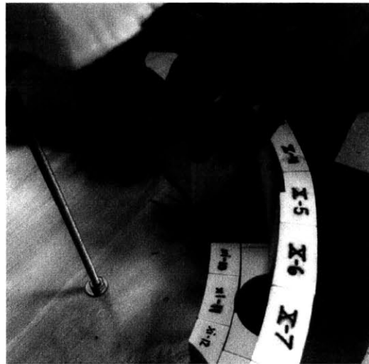
Figure 3.5: Image of the labeled blocks for courses 10 and 11 during construction
