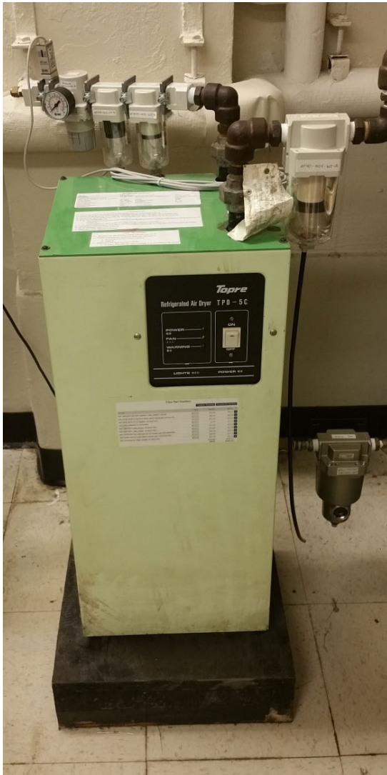
(a) Stage 1: Refrigerated air dryer with progressive filtering to dry the air.
