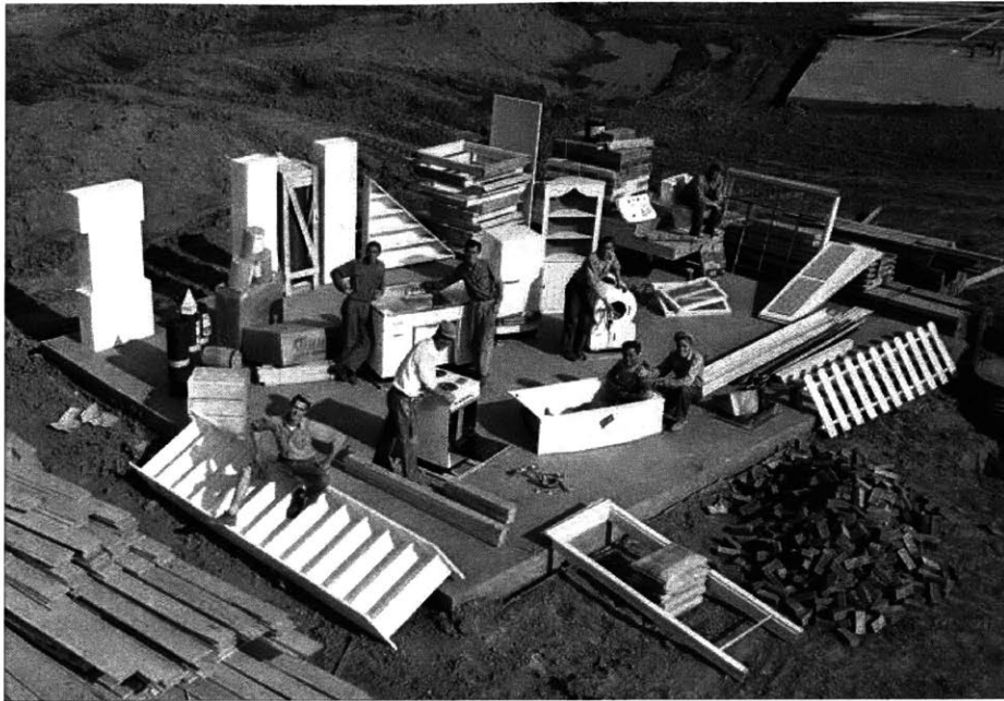
Every part of the house came prefabricated, even the stairs and fencing (Library of Congress).
