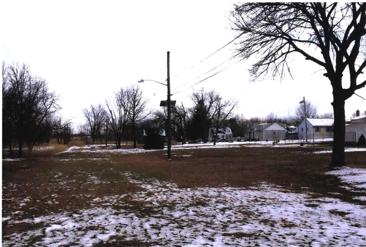
Figure 5.2: Where homes once stood, there is fresh soil and seed from demolition and ecological restoration work. The homes on the right are just out of the flood plain, and were not considered for buyouts. Photo by author.
