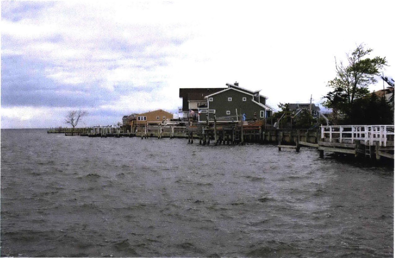
Figure 5.15: The Lindenhurst shoreline is densely developed with homes. The barrier island, barely visible in the background, provides protection from wave action. Photo by author.
