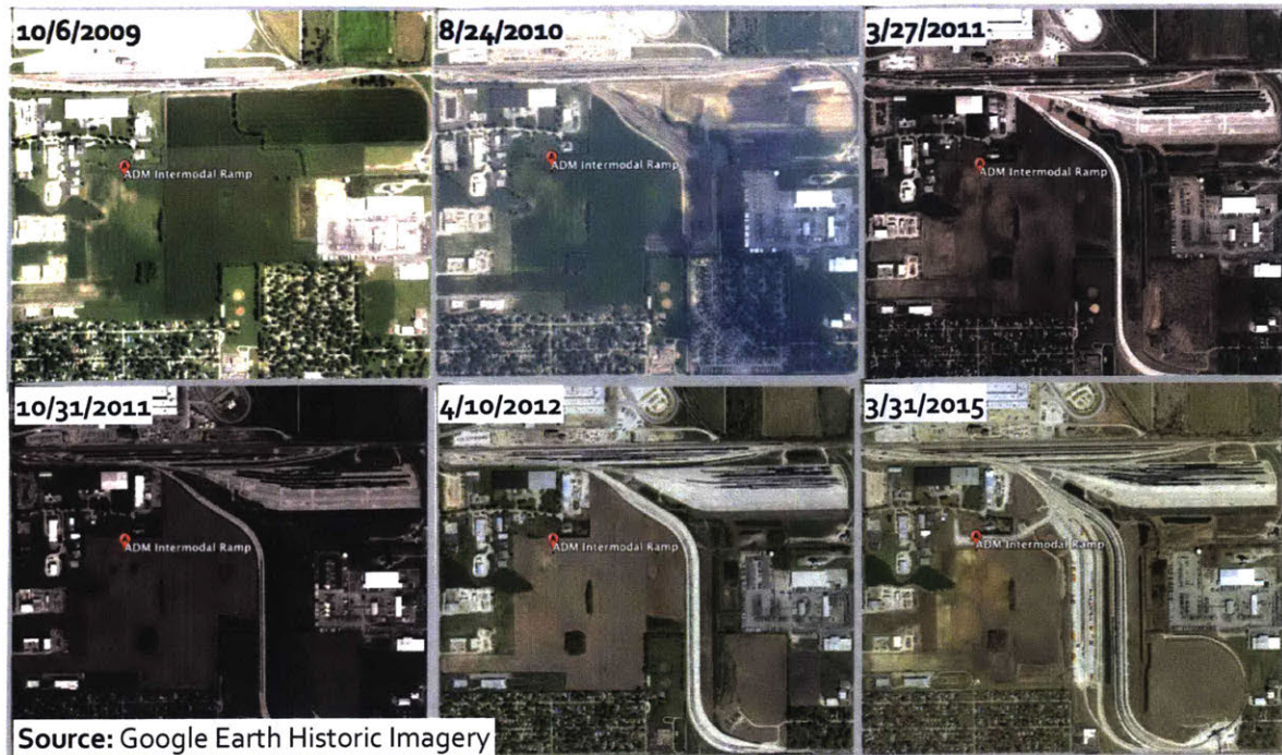
Figure 1—2: Time-lapse aerial imagery of the construction of the ADM intermodal ramp, from 2009 to 2015. Image Sources: Google Earth Historic Satellite Imagery.
