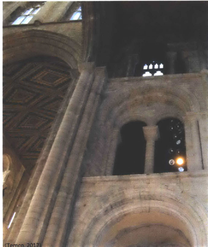
(b) Tower Pier
