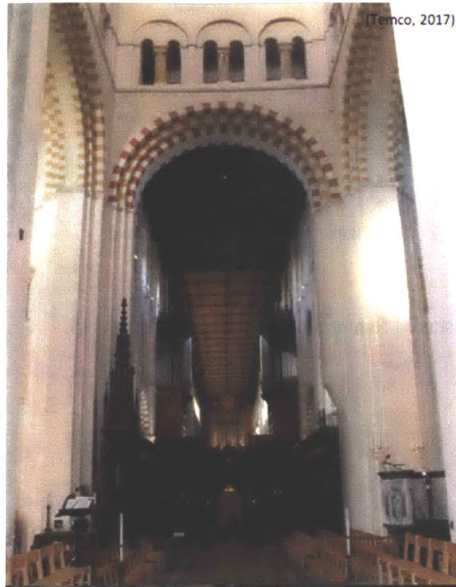
Figure 36: St Albans Central Tower Piers
