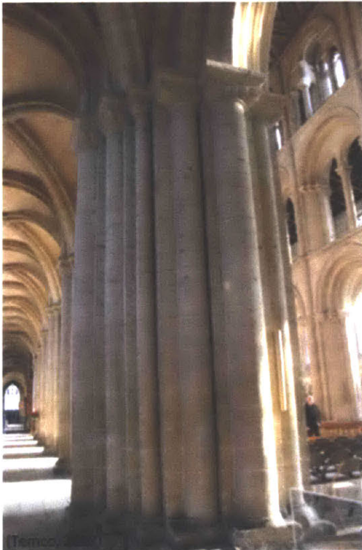
(a) Nave Pier
