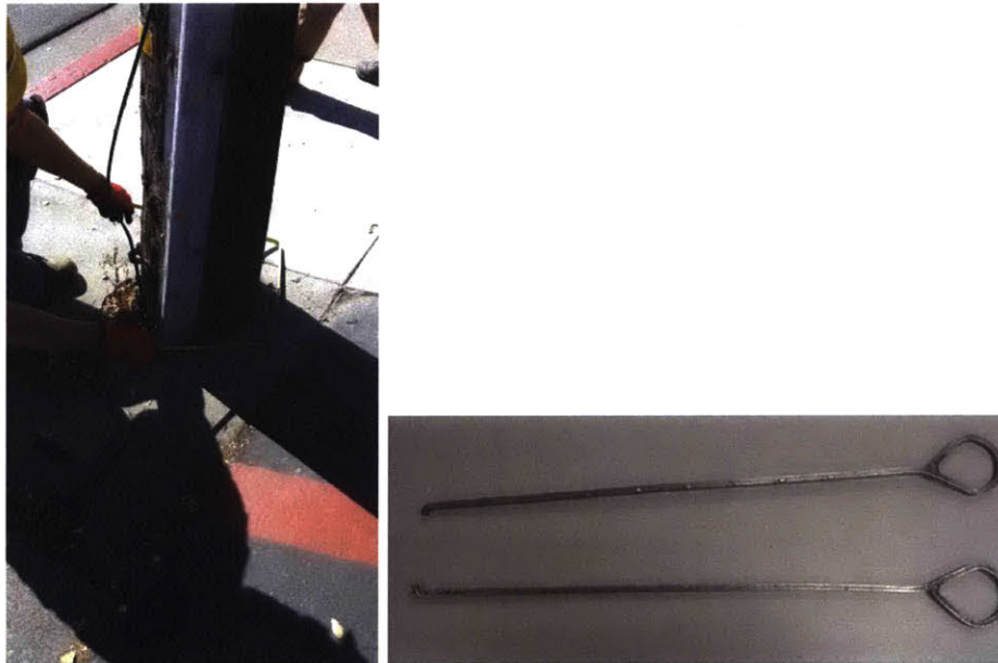
(a) Measuring circumference of pole (b) Instrument for measuring shell thickness and internal decay
