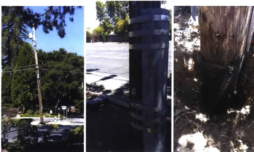
(a) Utility pole in San Francisco Bay Area (b) Structural reinforcement (i.e. stub) (c) Chemical treatment applied to poles
