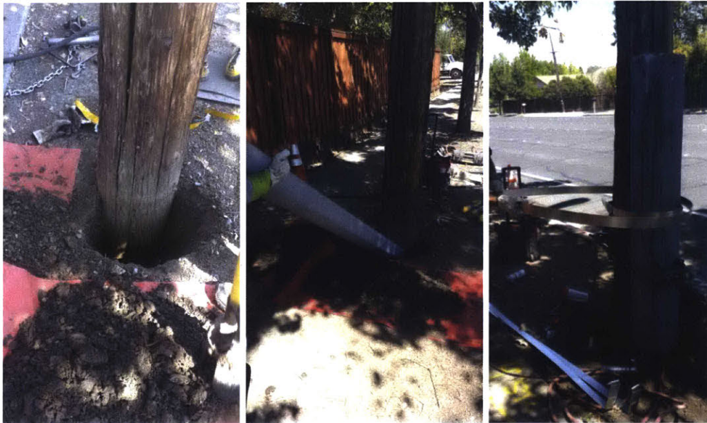
(a) Excavation for placement of steel stub (b) Placement of steel stub at rejected pole (c) Placement of bands to affix stub
