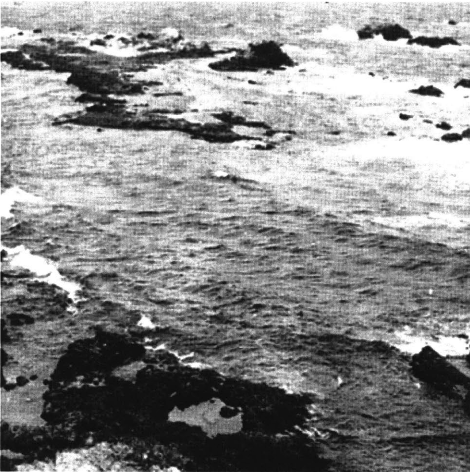
Historic image of Neft Dashlari's foundations
