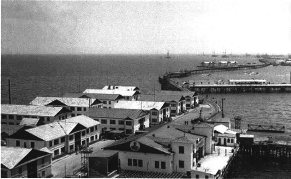
Historic image of Neft Dashlari's foundations
