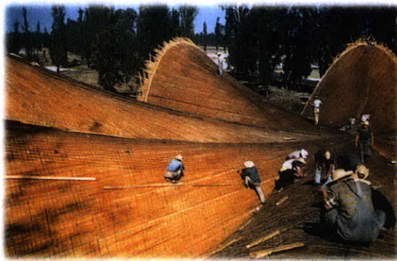
Fig. 4.7 Construction – Stave: Candela Formwork. | Fig. 4.8 Construction – Sheet: Fuller-Moore Plydome.
