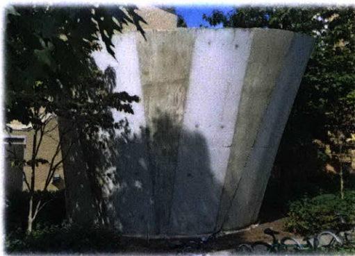
Fig. 2.23 Cast-in-Place Forms: Stata Center.
