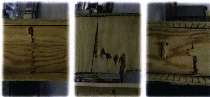
Fig. 5.12 Failure Modes: (a.) GEN.1_Panel, Control; (b.) GEN.0_Box, Kerfed; (c.) GEN.1_Panel, Kerfed. Web controlled failure at L/2; Web split at L/2 transfers to indexing; Web failure at L/3 at plug.
