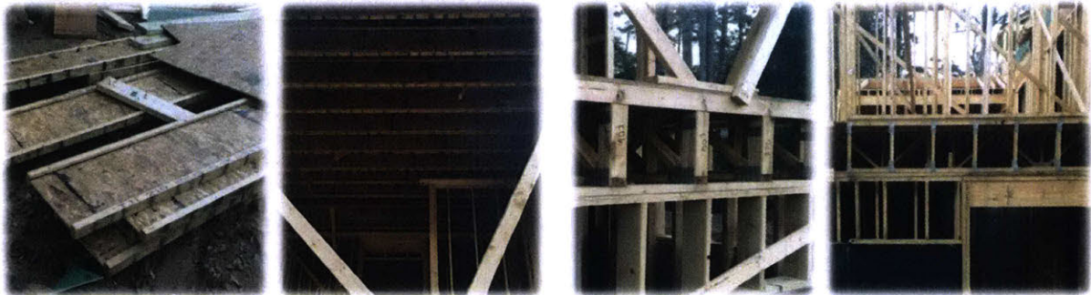
Fig. 4.1 Construction – Conventional: I-Joists. | Fig. 4.2 Construction – Conventional: Trussed-joists.
