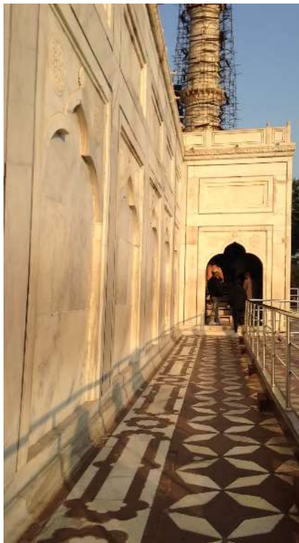
Fig. 12 Stairs onto the Plinth looking east
