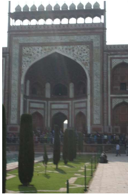
Fig. 32 Great Gatehouse north façade
