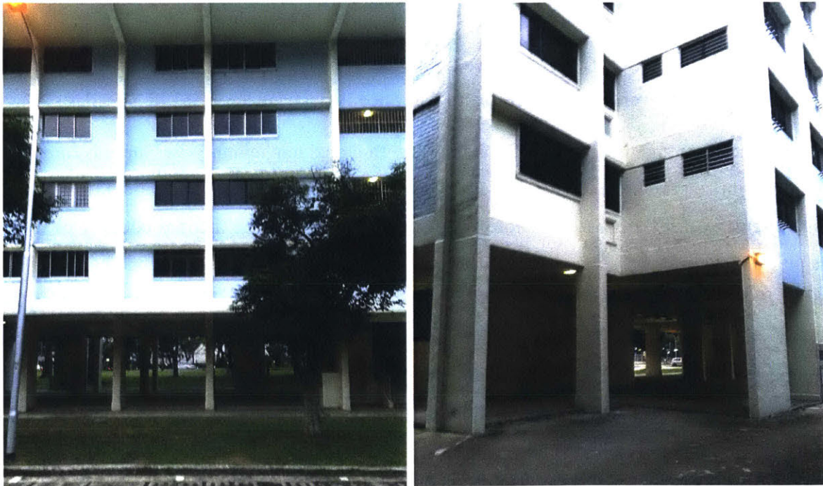
Fig. 1.4. Void decks, open spaces at the ground floors of public flats in Singapore.
