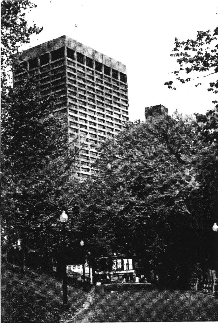
Fig. 44 Typical Boston Office Building, with identical facades despite different loads
