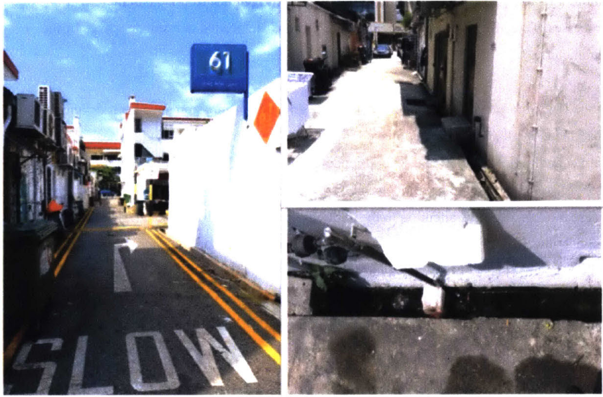
Figure 5.1. Outdoor breeding of the dengue vector Aedes aegypti occurs in clogged storm drain in Geylang, Singapore.
