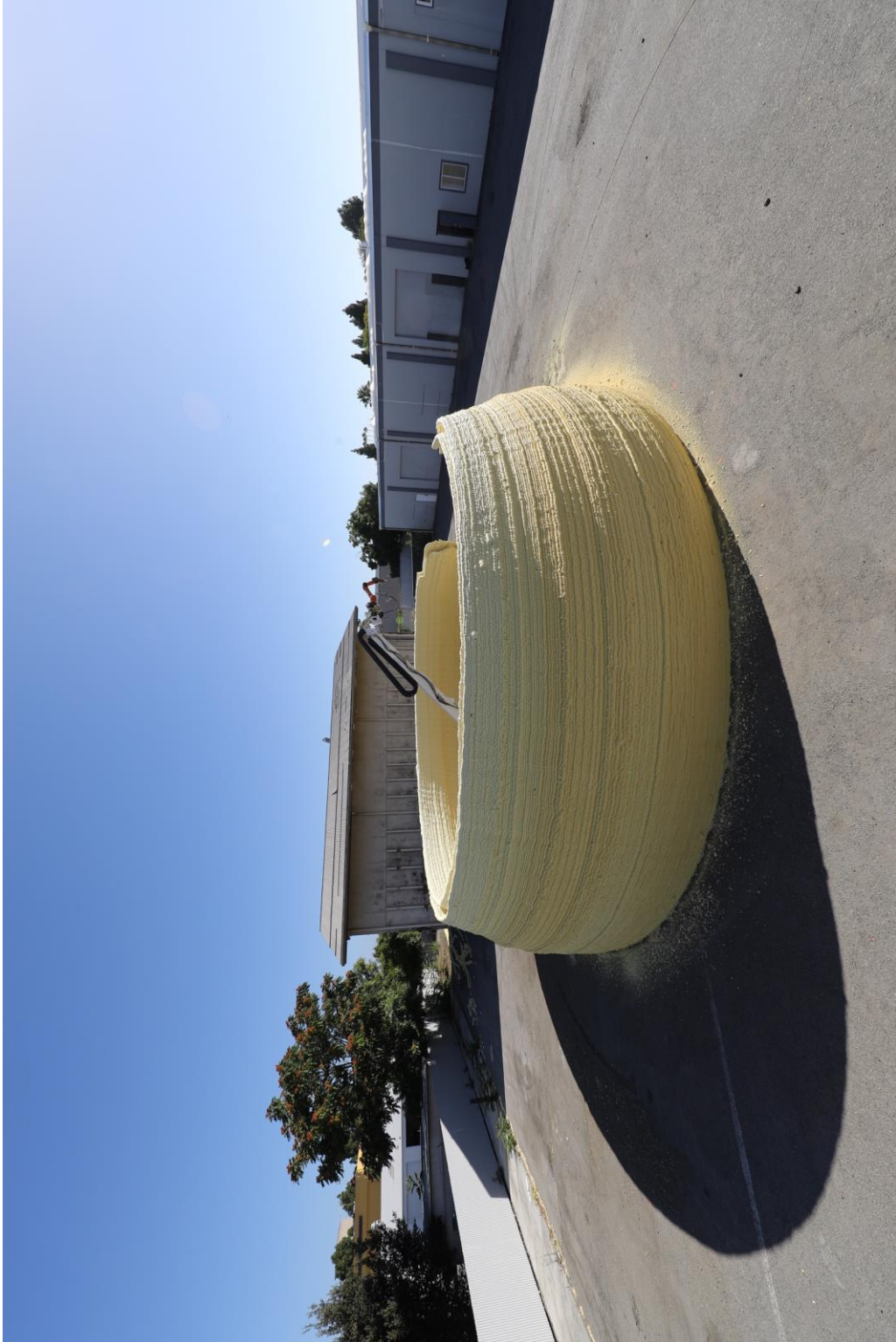
Figure 39: Completed dome. Image credit: Steven Keating.
