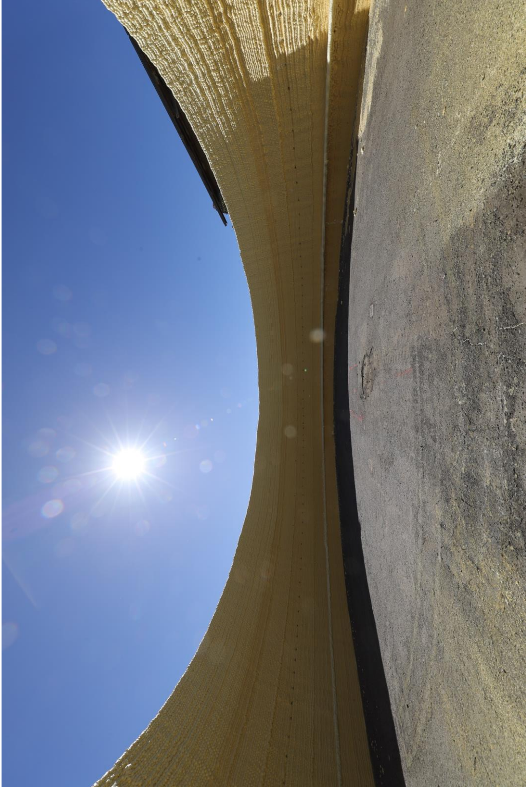
Figure 40: Completed dome, interior view. Image credit: Steven Keating.
