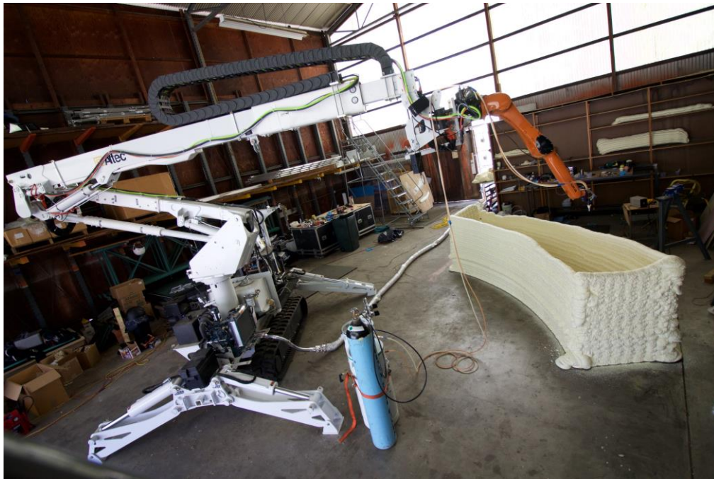
Figure 33: DCP with finished curved wall section. Image credit: Steven Keating.
