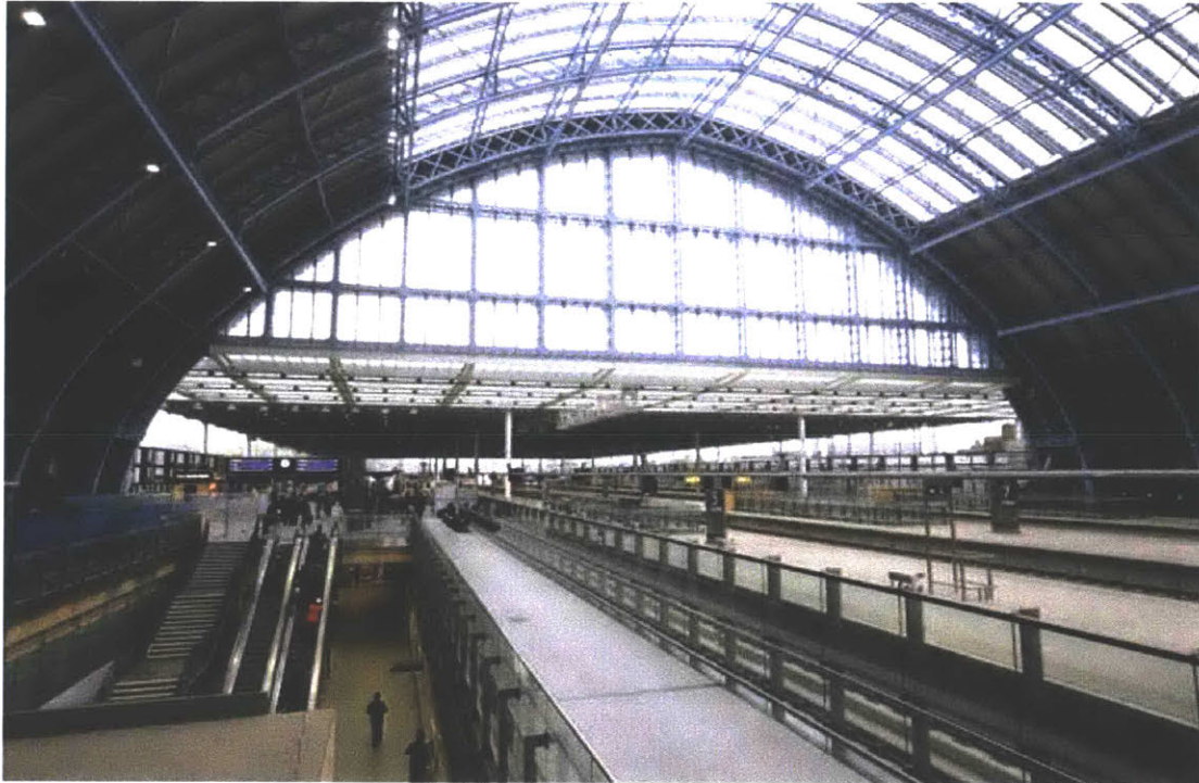
Figure 3-6. Refurbished St. Pancras Station: Barlow train shed, new train shed, platforms and below-ground concourse. ( The Guardian )
