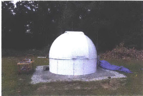
(m) 23 July 2014 - The completed dome.
