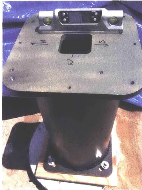
(f) 17 July 2014 - Leveling the metal pier.
