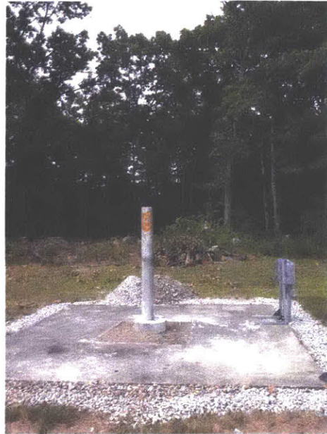
(b) 3 July 2014 - The finished concrete pad with draining trench.
