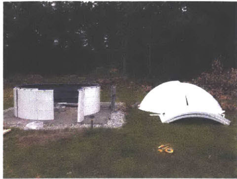
(e) 16 July 2014 - Laying out the dome on the concrete pad.
