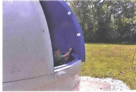
(j) 22 July 2014 - Tim Brothers attaching the dome to the dome rings
