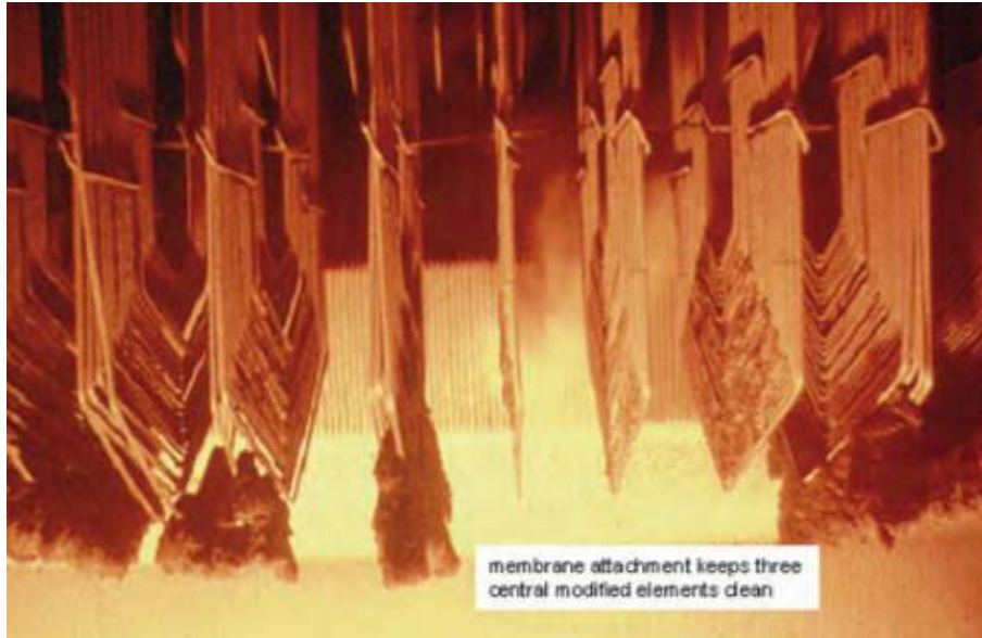
Figure 1-1: Ash fouling on superheater tubes in a coal-fired power station [14]. The fouling deposits are the fluffy layers on the bottom of the superheater tubes.
