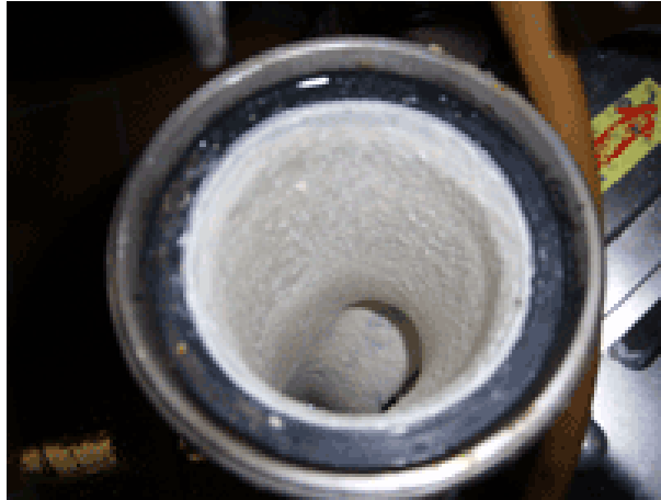
Figure 2-3: This image shows the reaction fouling of milk pipe in a milk-processing plant [62].
