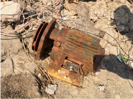
Figure 41: Rusted Pump Seen in the Little Rann of Kutch
