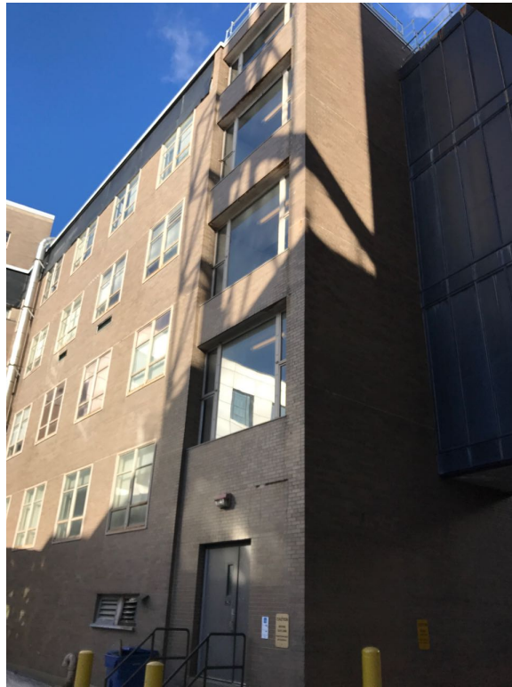
Figure 3-1: Photograph of the stairwell exterior in Building 35 at MIT used in the full scale experiment.
