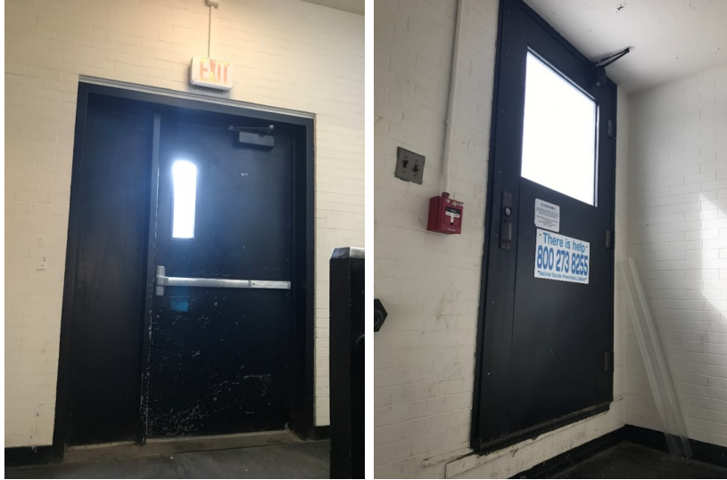
Figure 3-4: Photographs of two openings connecting the stairwell and ambient. A bottom door(left) on the ground floor is open during the experiment and a top door(right) leading to the roof is left open.
