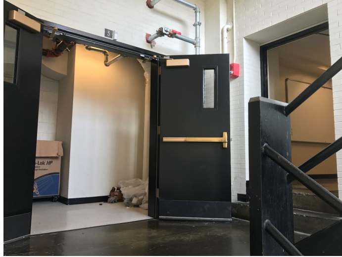
Figure 3-3: The photograph of the doors connecting corridors and the stairwell.
