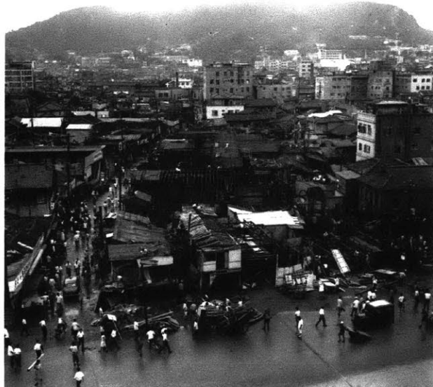
execution of the emolition order, 1967
