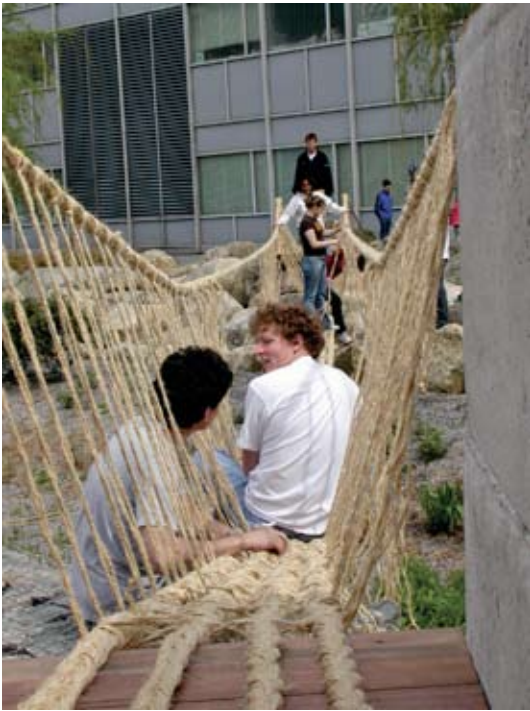
Figure 4. Students installing the Chaka Stata. Estudiantes instalando el Chaka Stata.
