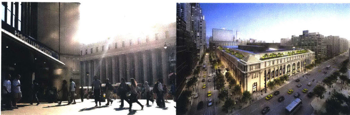
Exterior of James Farley Post Office today (left) and rendering of the future Farley-Penn Station (right), Rendering: Courtesy of Skidmore, Owings & Merrill (SOM)
