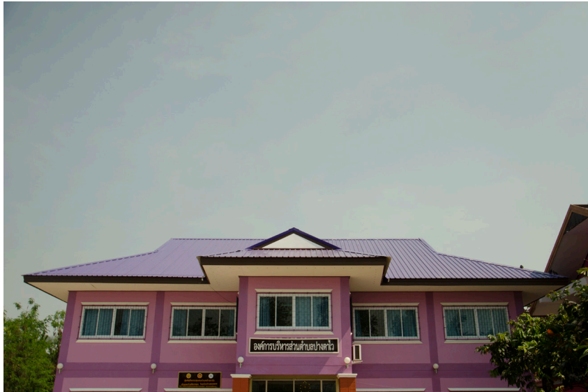
Figure 4-2: Sub-District Administrative Office
