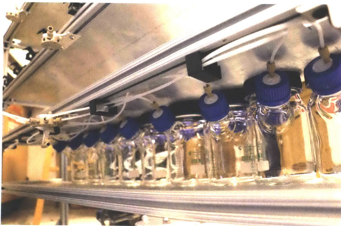
Figure A2.7: Bottles to serve one valve with nitrogen lines installed. Note that reagent lines have not yet been installed in this photo.
