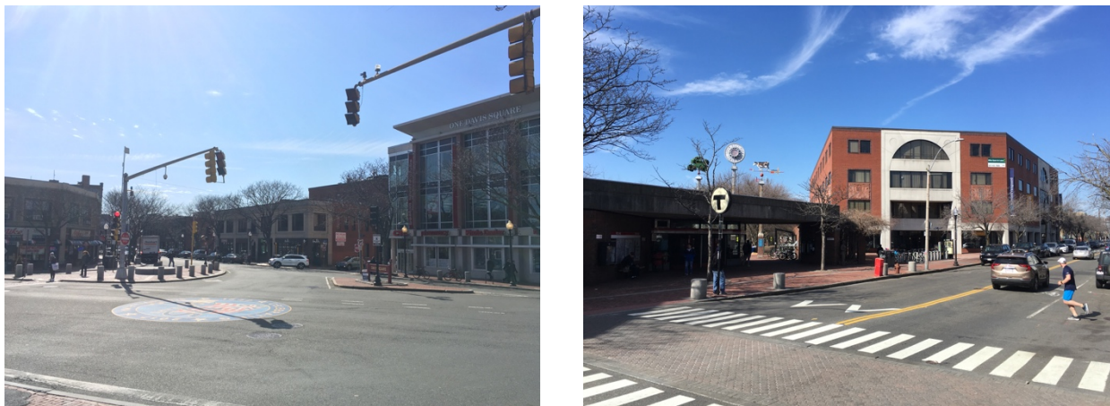
Figure 6: Davis Square in February 2018 (Left: a view across the square with One Davis Square on the right and Elm Street opposite. Right: the Harvard Vanguard building on the right and Red Line station on the left with the bikeway behind it. Source: the author.
