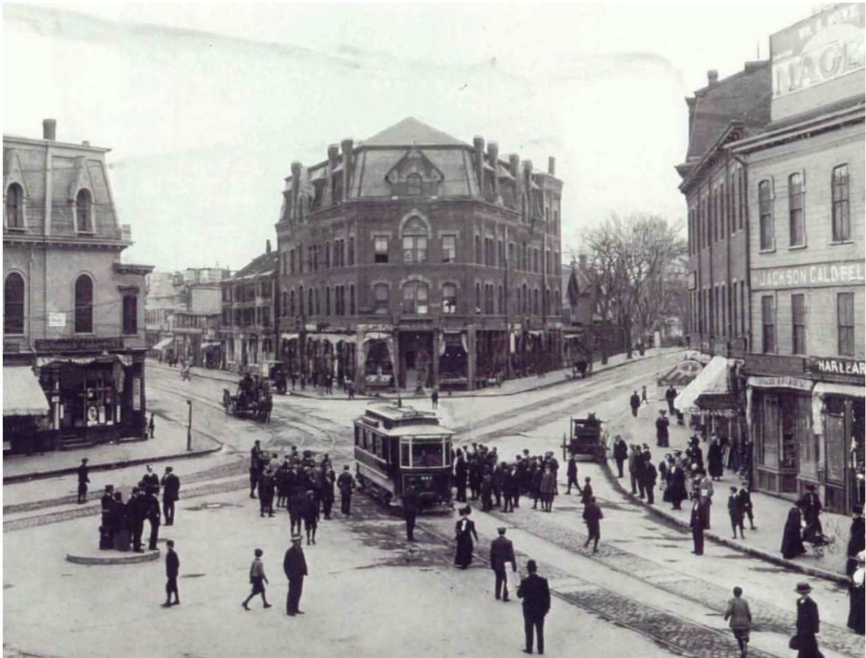
Figure 14: The intersection of Bow St and Somerville Ave in Union Square in the 1920s. Source: OSPCD. 138
