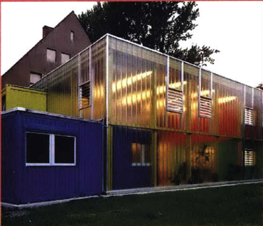
Time-Based Prefab Structures bed by night, Hanover (bed-by-night.de)
