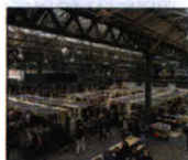
Bully Installation Near Spitalfields Market, London (Credit: M&P)
