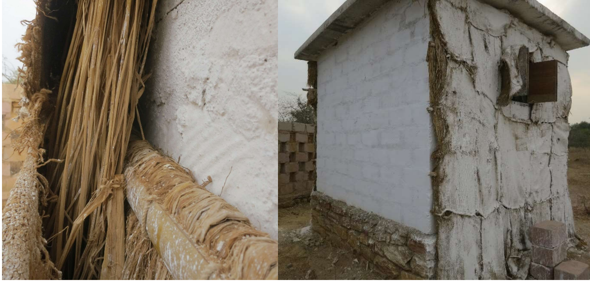
Figure 54: Straw Insulation on Chambers 3 and 4 (January 2018)
