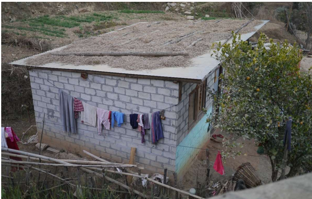
Figure 95: Metal sheet roof with straw covering (Chitlang, Nepal)
