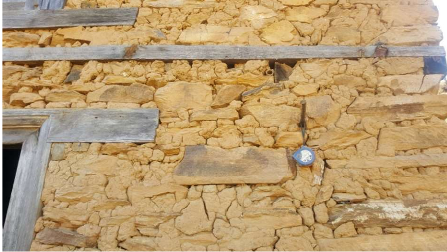
Figure 78: Timber-reinforced Stone and Mud construction, Chitlang, Nepal
