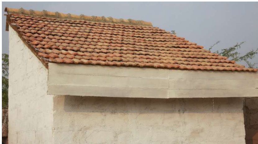
Figure 49: Mangalore Tile Roof, Test Chamber 2
