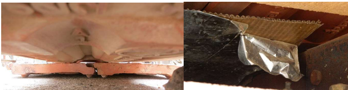
Figure 47: Left: Overlap of Mangalore tiles showing unfilled space (credit Vadim Kuklov), Right: Radiant barrier as applied in Ramdev Nagar homes, January 2017
