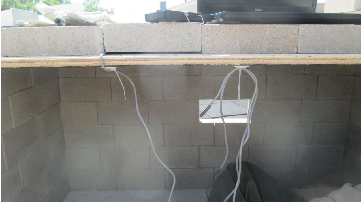
Figure 3: Dry-fit assembly prior to addition of waterproofing
