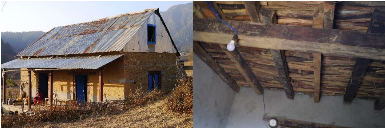
Figure 82: Chitlang rural reconstruction (Completed project), Right photo courtesy of Vadim Kuklov
