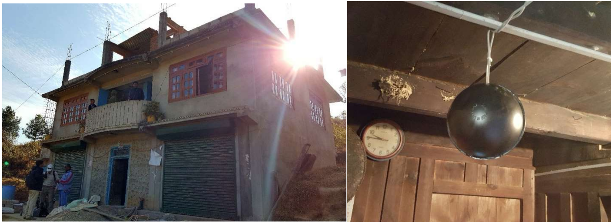
Figure 89: Left: RCC Home serving as the Hunnarshala field office, Right: Radiant Ball installed in the Traditional home
