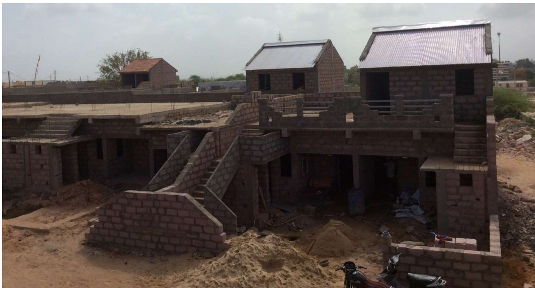
Figure 63: Ramdev Nagar homes under construction, Summer 2016 (Photo Credit Tejas Kotak)
