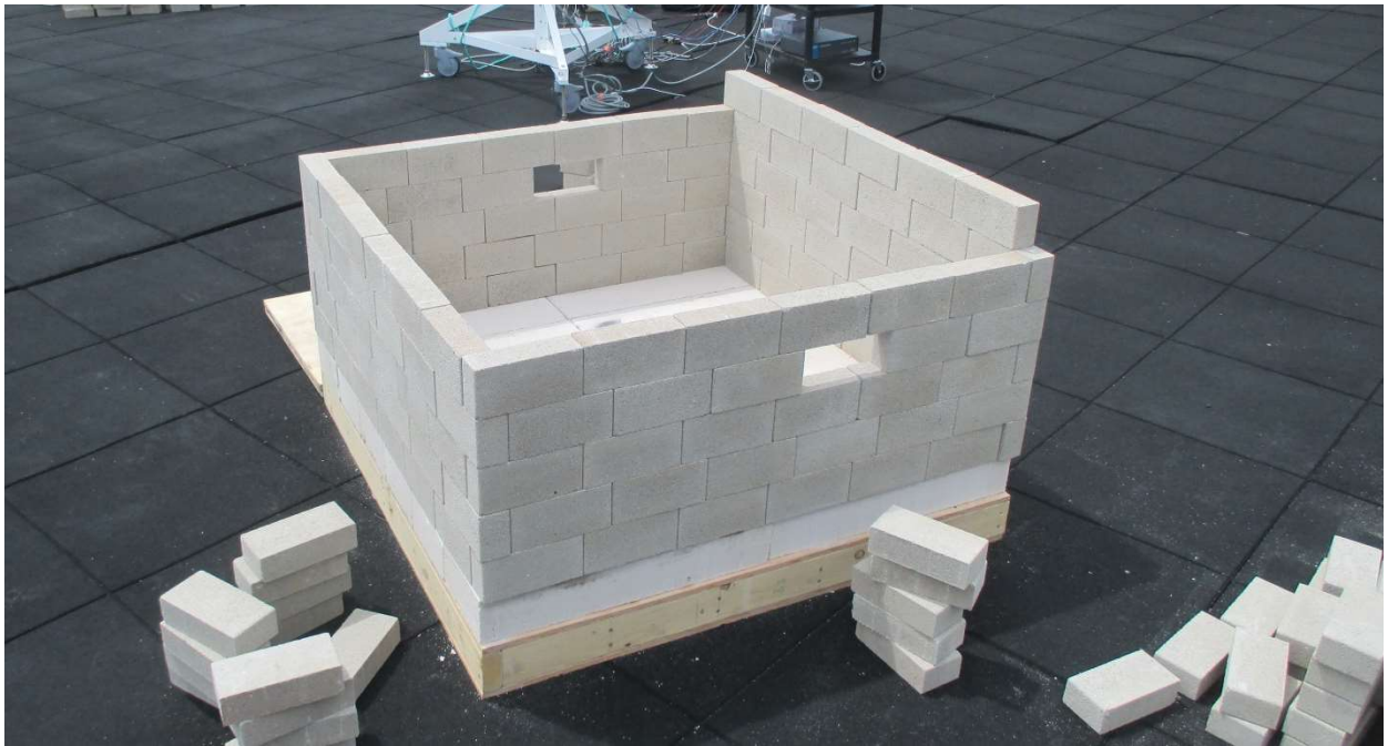
Figure 2: Test chambers midway through construction
