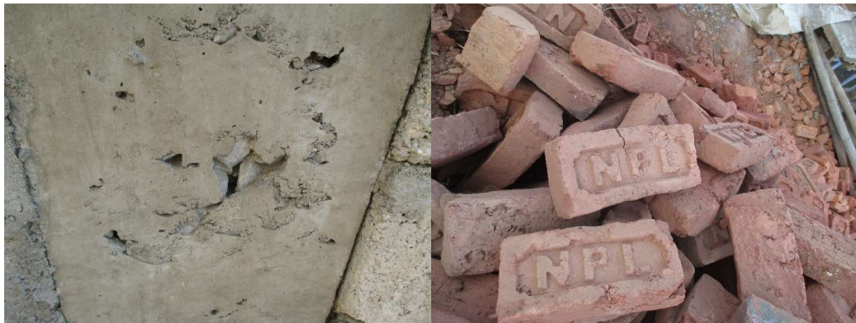
Figure 84: Left: RCC column, Right: Brick delivery (Chitlang, Nepal)
