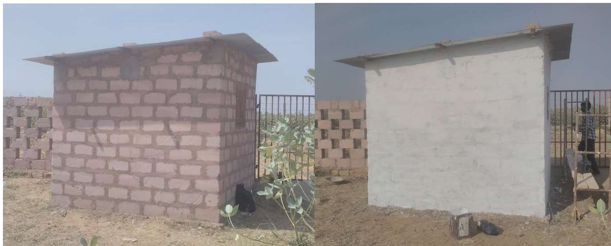
Figure 42: Chamber 1 before (left) and after being painted (right). Photos courtesy of Pradip Rangani, Hunnarshala.
