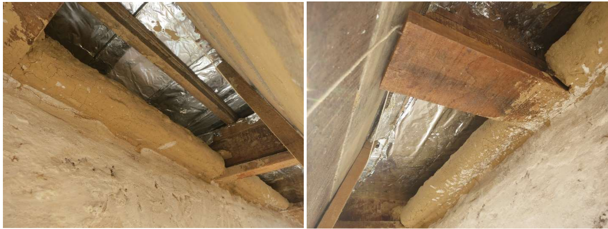
Figure 48: Directly applied radiant barrier (left) and radiant barrier applied to cardboard (right)
