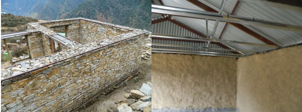
Figure 81: Chagam nunnery reconstruction project (construction in progress, January 2017)
