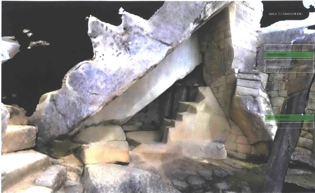
Screenshot 5. Photosphere view, photograph layer turned-off, 3D Scan layer turned-on
