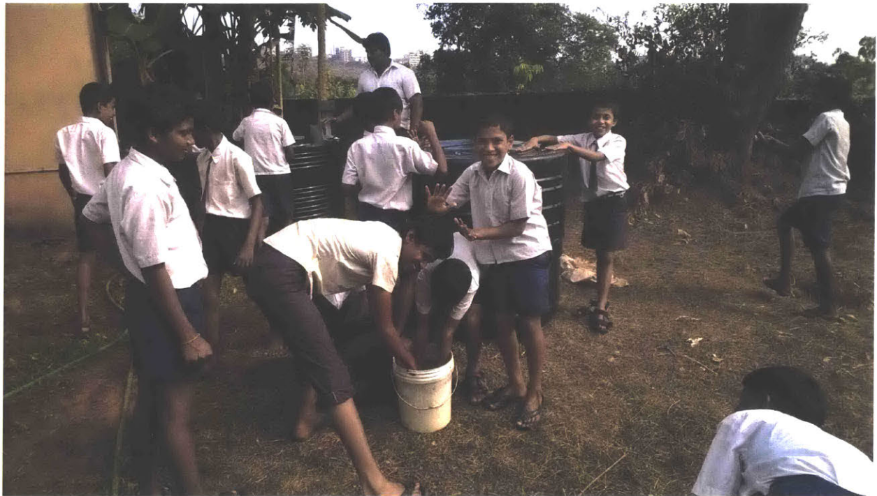
Figure 4: Constructing a biogas plant in another school
