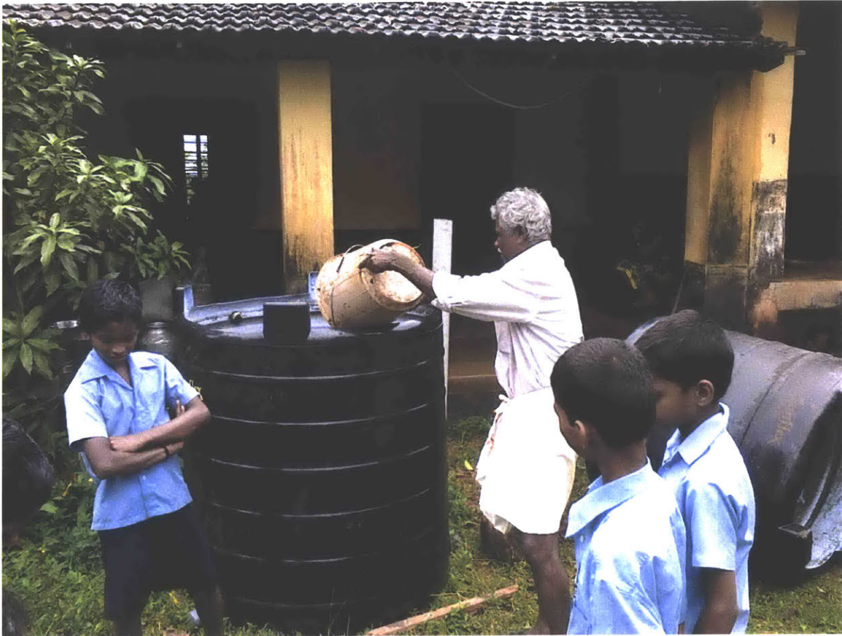
Figure 2: Assembling the biogas plant
