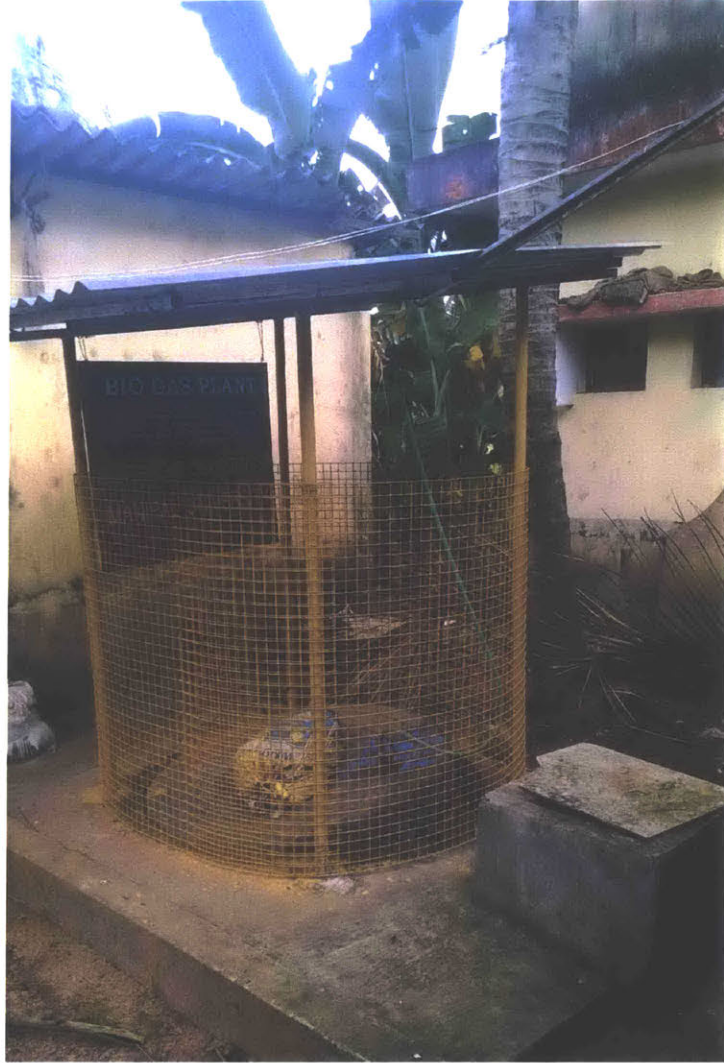
Figure 11: An 2 m 3 underground plant at an orphanage with feeding chamber and shed
