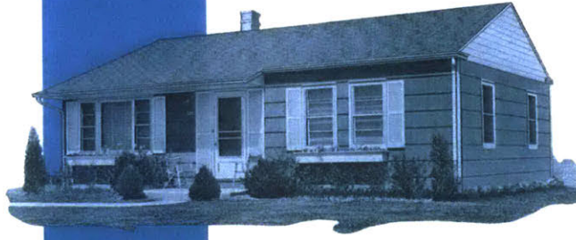
A 34° partial overhanging cornice, two pairs of outside window blinds plus a pair of 3'0"x5'8" door blinds, and two assembled flower boxes with ornamental iron brackets add immeasurably to the clean-cut lines of this modern home.
