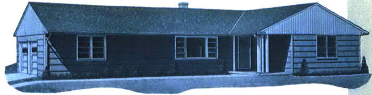
The long, flowing lines of this distinctive home are created by a wide overhanging cornice across the front, tying the 24'0" x 24'3" two-car garage and home together. 1x8 V-joint siding is used effectively on gable ends. The 24'3" front gable extends over the front bedroom to form a 6'x12' wood columned porch.
