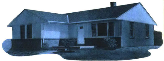
This conventionally-styled home has a 34" overhanging cornice over entire front, rear and sides of the front bedroom extension. Brick veneer and 1x8 V-joint siding combine to present a striking appearance.
