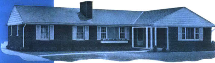
This well-proportioned ranch-style home, typifying Pease flexibility, features a 24'0" x 24'3" two-car attached garage with doors at the rear; a 6'x12' front porch, with 24'3" gable over front bedroom and a Panorama window panel in place of 2 single windows in bedroom. Brick veneer is obtained locally and field applied.
