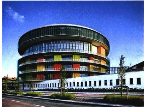
Figure 3: Malmö University Hospital, Sweden xxiv
