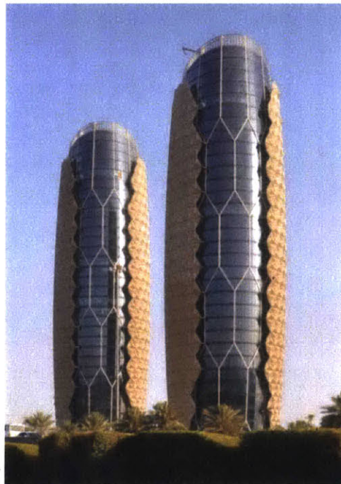
Figure 12: Al Bahar Tower Hexagonal Frame (Arup, 2013)
