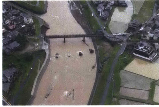
Figure 2- Hito River Railroad Bridge collapse by flooding and scouring in Japan after Typhoon Nanmadol in 2012 [7]
