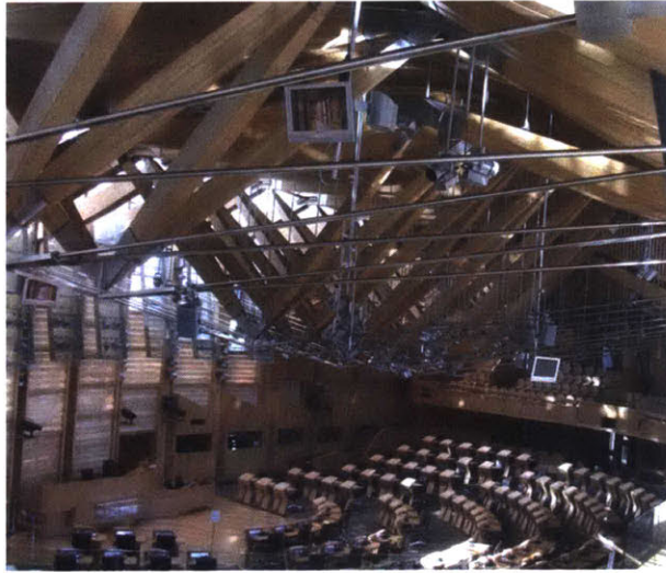
Figure 4: The Scottish Parliament building is an example of a steel and timber roof design [8]
