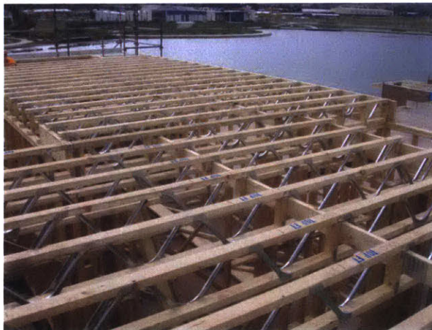
Figure 5: An open web joist [9]
