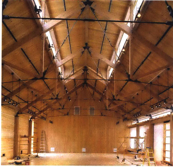
Figure 6: The Depot designed by Bridgeport Design Group [10]
