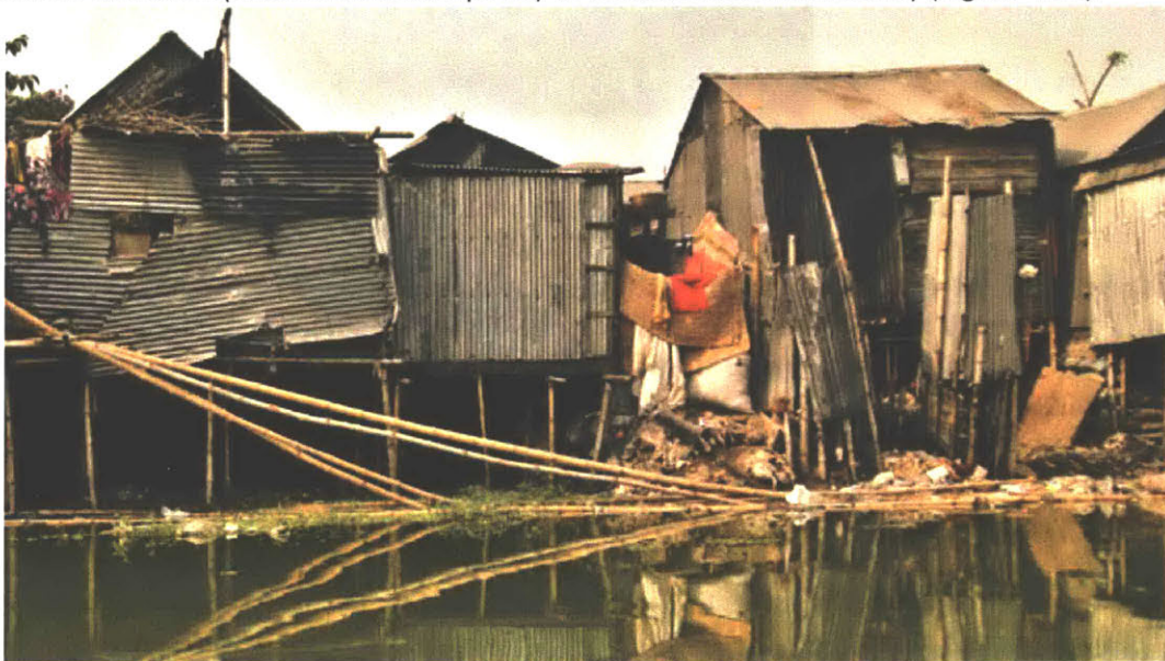
Figure 4.15. Elevated dwellings in informal settlements inside Dhaka's western embankments.
