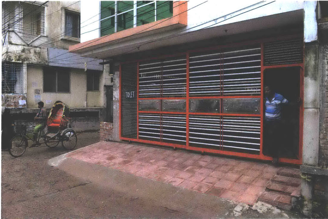
Figure 4.14. Elevated apartment block with ground floor parking inside Dhaka's western embankment.
