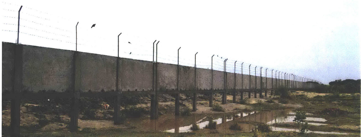
Figure 4.20. Enclosure walls deployed by private land developers in eastern Dhaka. By leaving the bottom of the walls open, developers allow the sand slurry used to elevate their land to spill onto adjacent land and waters, rendering them unfit to provide the fishing and farming livelihoods on which residents of peri-urban areas rely.
