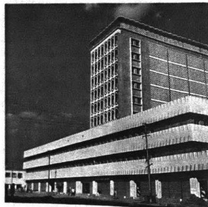
EPWAPDA Headquarters, Dhaka
