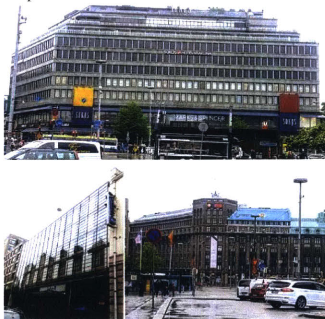
Figure 6.2.1 Helsinki's Consumer Cooperatives. North, East and West around Helsinki's main center and rail station, you find anchor businesses like the sleek Radisson Blu hotel (left), a branch and prominent signage of OP bank (right) which is Finland's largest financial institution, and SOK's Sokos Department store, restaurant and hotel complex, which includes the flagship Marks and Spencer's (top). All of these businesses are consumer-owned Finnish cooperatives, whose profits go to their user-owners. Only in Finland are Radisson and M&S held as coops.
