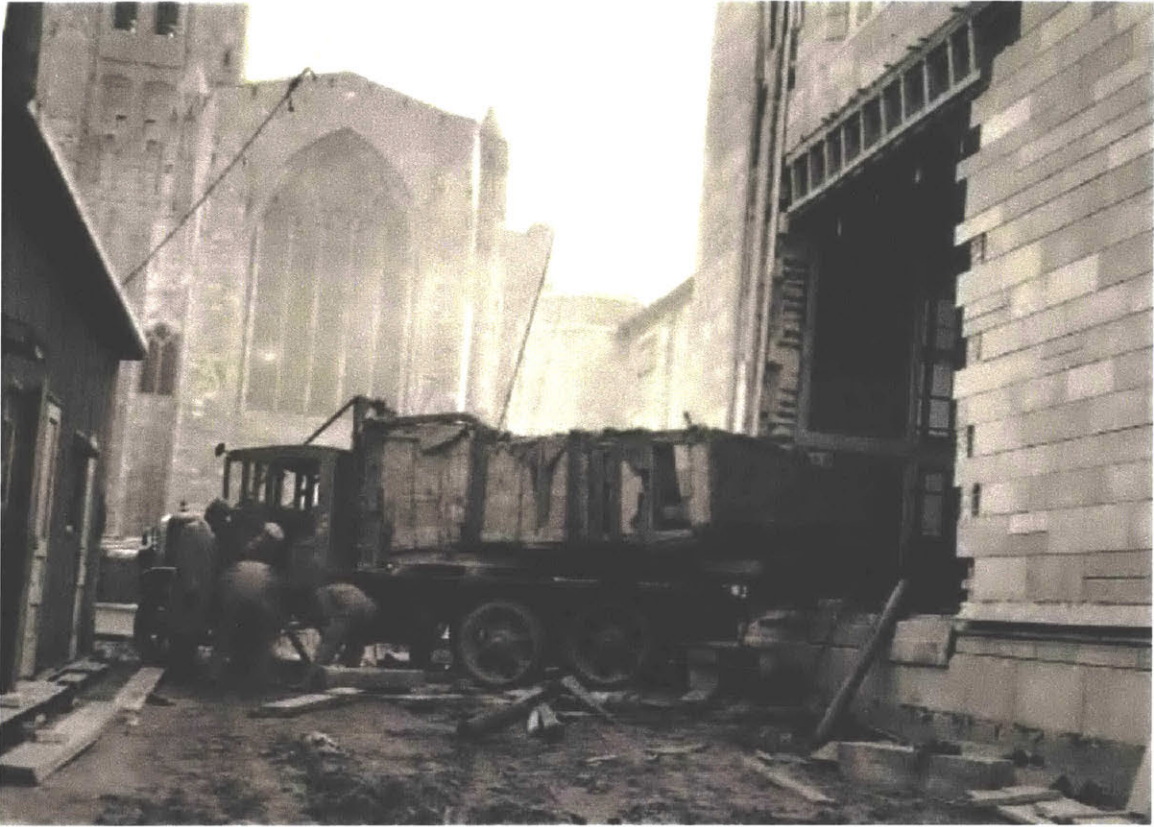
6.72 A truck bearing the bull backs up towards the Oriental Institute building. The bull was then lifted and hauled in to the building through the hole in the wall. In the rear, we can see the Rockefeller Memorial Chapel. Source: OIA. Courtesy: O.I.
