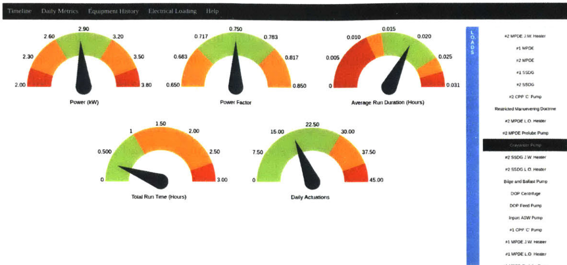
Figure 1-5: NILM Dashboard metrics indicating healthy gray water pump operation.
