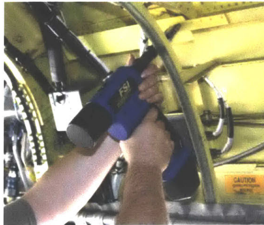
Figure 2: Manual overhead riveting[4]
