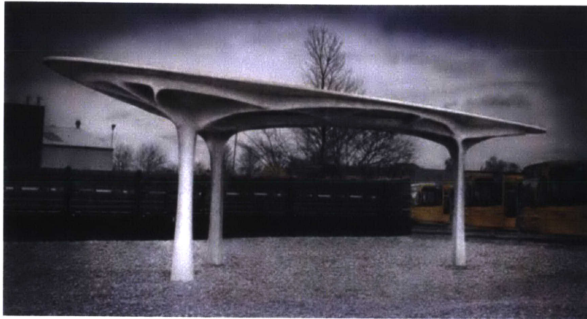
Fig.2-5 Finalized prototype concrete shell structure
