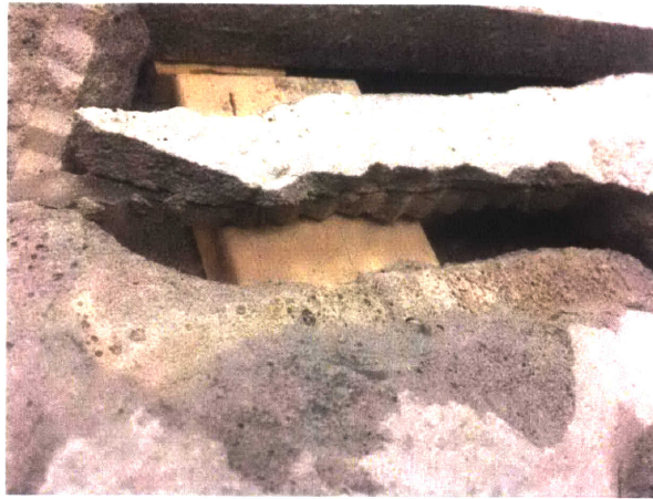
Fig.5-2-3. Polished surface of contact between the steel and concrete
