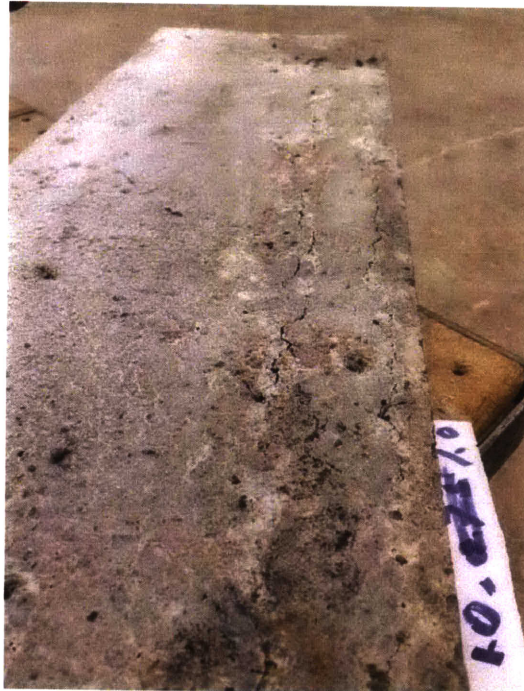
Fig.6-2 Initial cracking in the beams
