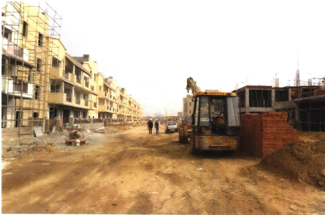
On the left of the photo is a row of houses with nearly-complete facades. The type of bricks that lie under the plastered and painted facades are shown on the right of the photo. Photo: Mohamed Ismail
