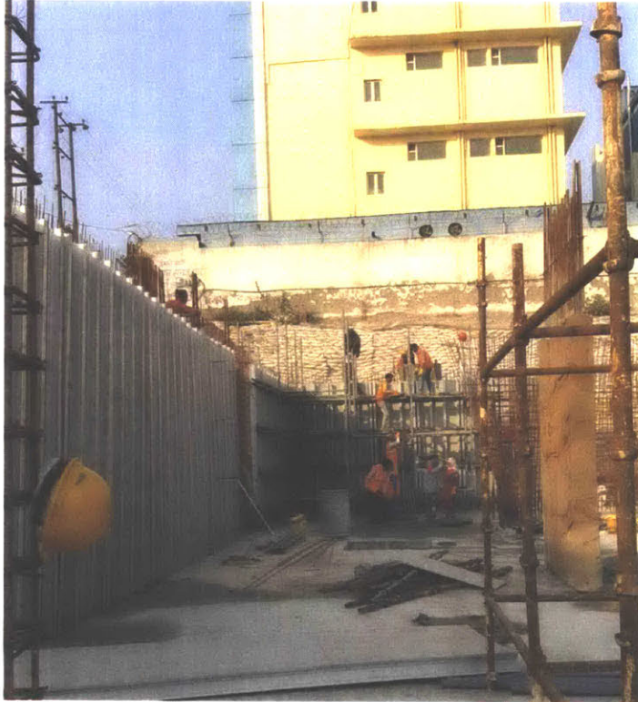
The people at the top of the scaffolding are pouring concrete into the formwork. Two hard hats are visible, but note that the majority of workers are not wearing them. Photo: Abigail Anderson Site 2
