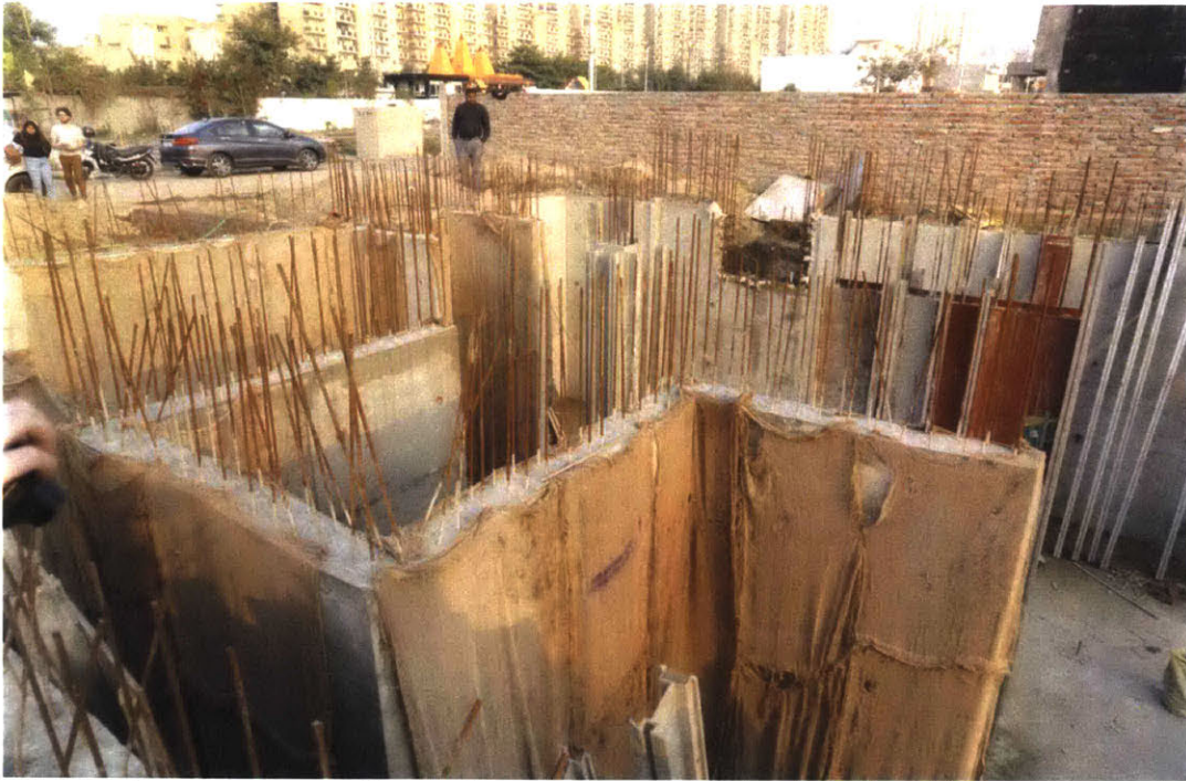
Burlap covers the concrete walls as they cure to reduce moisture loss and cracking. Photo: Mohamed Ismail
