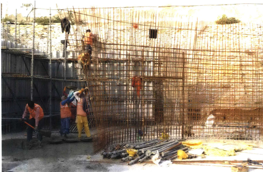
The end of the concrete-pouring bucket brigade: workers carry concrete on their heads and then lift it up to the person at the top of the ladder, who slowly and carefully pours it into the formwork. Photo: Mohamed Ismail
