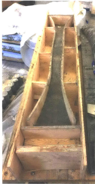
Demolding of the bent wood beam. Photo: Yan Liu.
