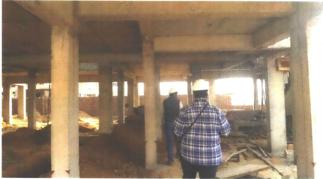
The formwork patterns used for pouring the first-level floor slabs are visible on their undersides. Plywood of various sizes is evident. Photo: Abigail Anderson
