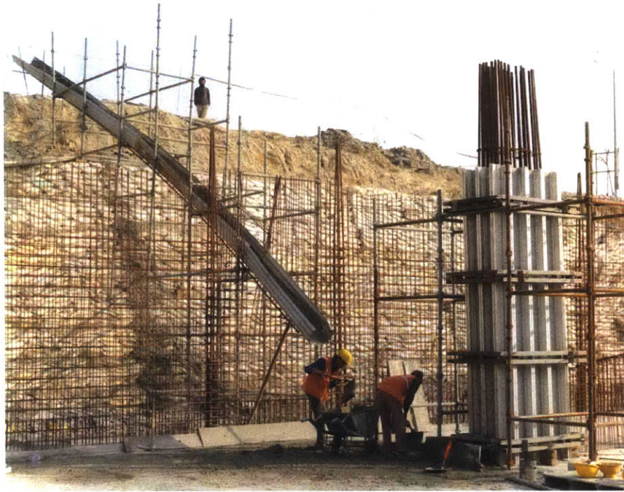
Concrete is mixed at the top of this hill, near the site entrance, and then shoveled into this chute. At the bottom, a wheelbarrow collects the concrete and then a worker wheels it to the part of the site where it is needed. Photo: Mohamed Ismail
