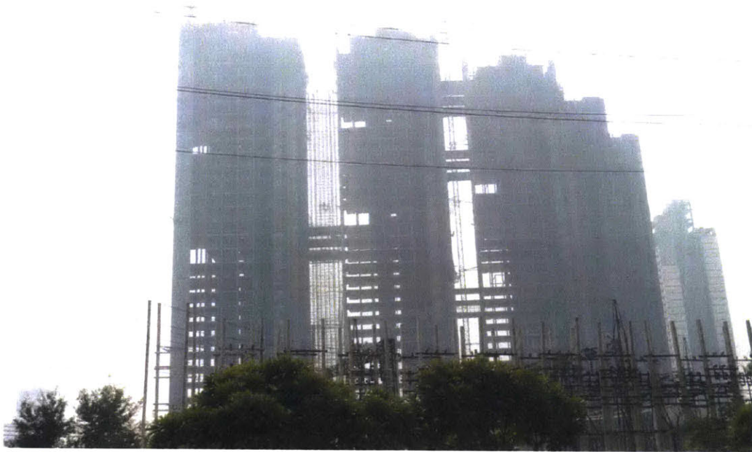
Massive tower cranes and thirty-story scaffolding support the construction of these reinforced concrete buildings. Note the several bridges between towers, and the thick smog present in many major Indian cities. Photo: Mohamed Ismail
