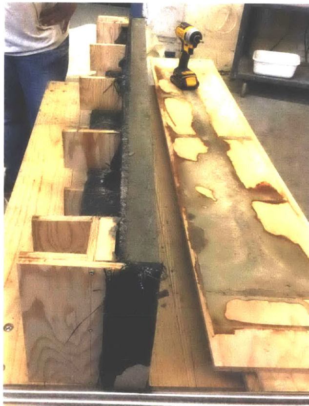
Removal of the fabric formwork. Photo: Yan Liu.
