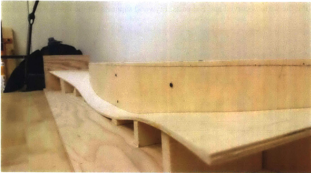
Attaching the flange supports to the curved pieces and the base
