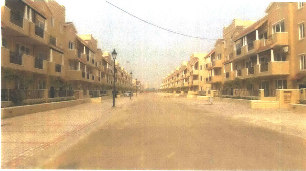
This street is nearly complete. Photo: Abigail Anderson
