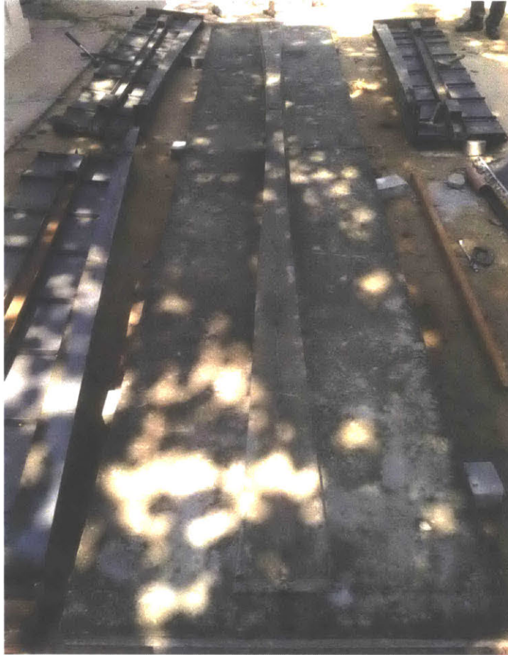
Figure 34: Full-scale T beam, constructed in Delhi by TARA, using rolled steel formwork (visible in photo). (Credit: Biswajit Swain)
