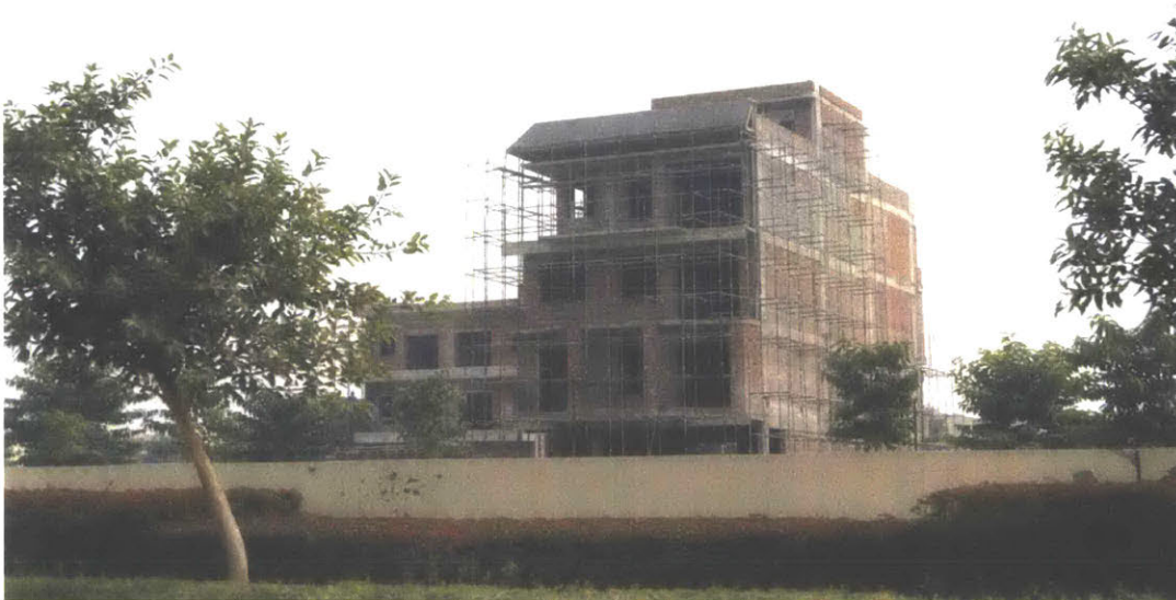
Smaller-scale construction projects are also common. This building uses a different type of brick for its exterior facades between concrete slabs and columns. Photo: Mohamed Ismail
