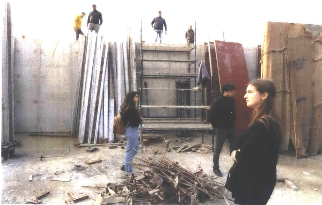
The second site, again by Harsh Vardhan Jain Architects, is a smaller residential project. Plywood formwork (red) and aluminum formwork structuring (silver) are visible. Workers on this site were resting (top). Photo: Mohamed Ismail
