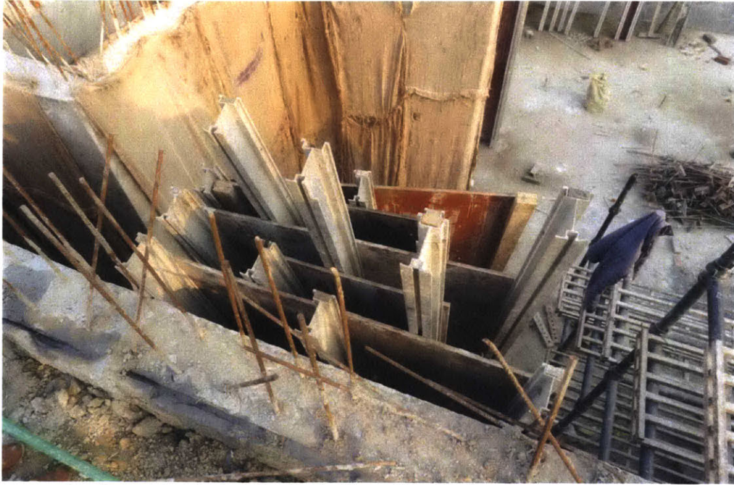
This site uses aluminum structuring that is similar to Site 1's, but the material touching the concrete itself is plywood instead of HDPE. Red sandstone, colored gray here from the concrete, is used along the outside of the foundation as waterproofing. This material would be expensive elsewhere in the world, but in this area, it is more common. Its porosity makes it a good waterproofing material. Photo: Mohamed Ismail
