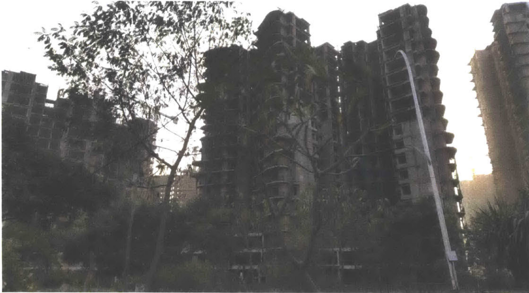
Tower blocks under construction in Delhi. Bricks, likely fly ash, compose the exterior walls on lower stories. Photo: Abigail Anderson
