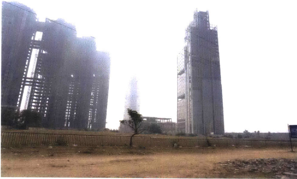
Figure 3: Massive concrete structures are emerging in open fields. (Credit: Ismail)
