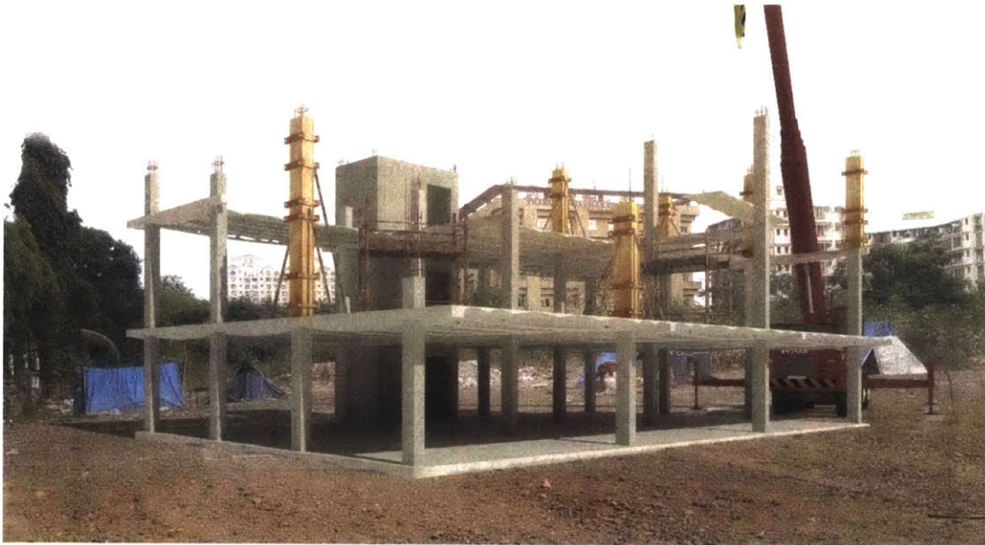
Figure 2: Computationally optimized slabs in Indian construction context (Credit: Ismail)
