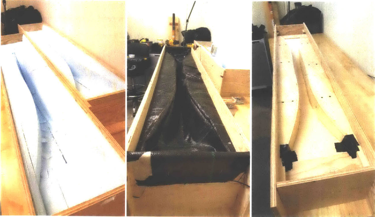
Figure 29: Milled foam, fabric, and bent wood final formworks
