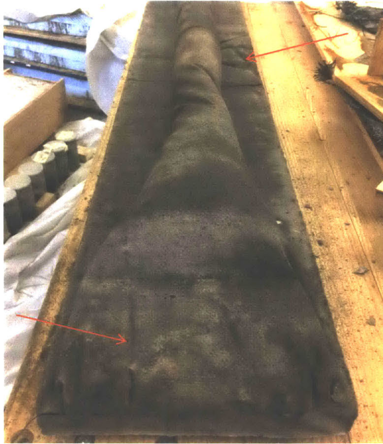
Figure 33: Evidence of wrinkles from fabric formwork
