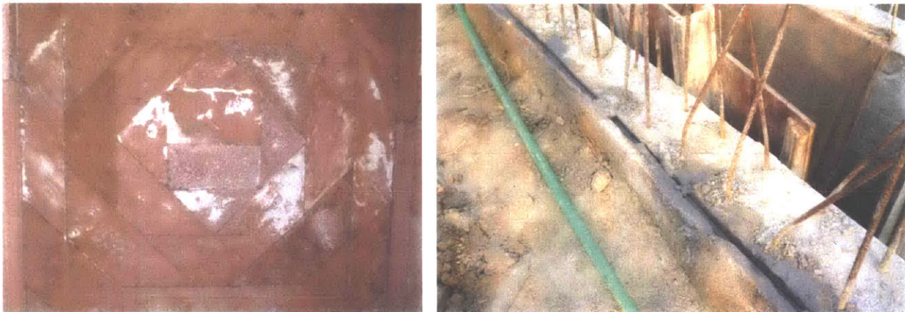
Figure 14: Red sandstone is widely available in northern India and has been used for both (a) flat domes (Credit: Anderson) and (b) waterproofing (Credit: Ismail)
