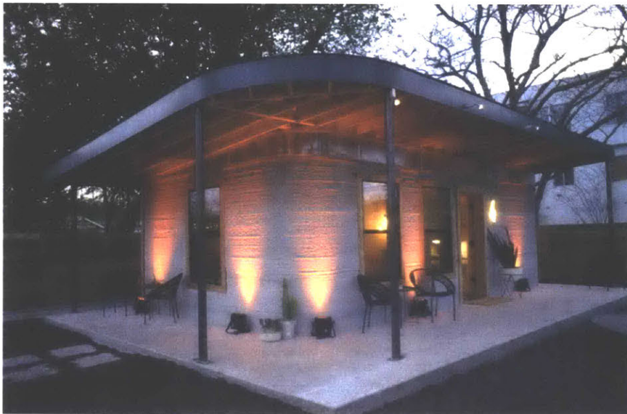
Figure 10: A 3D-printed home that costs only $4,000 (Credit: Bendix 2019)
