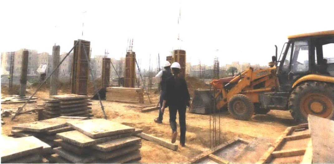
At EMAAR's Emerald Hills site, we saw large-scale residential construction at several stages of the construction process. In this part of the site, still in the early stages of construction, columns are being cast. Rebar and stirrups are visible on the right, and a completed ground-level column is visible on the left. In the background on the left is a row of nearly-completed homes that are part of the same site. Photo: Mohamed Ismail
