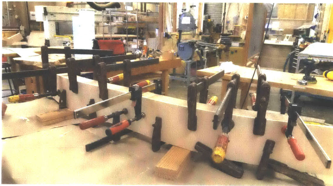
Clamping 3 layers of 1/8" plywood to the MDF form, with wood glue in between.
