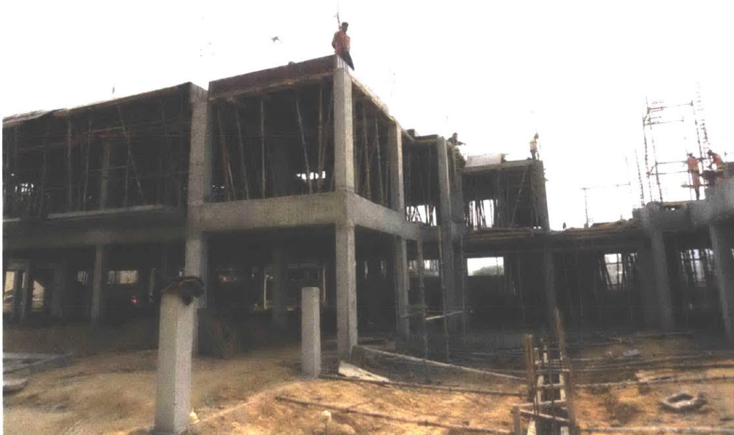
Concrete slab construction with shoring supporting second-level floor slab formwork. Photo: Mohamed Ismail
