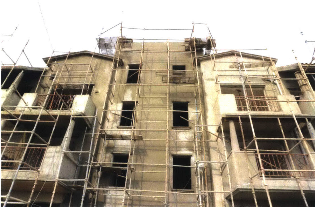
The exterior facade in the process of drying, with scaffolding for workers still attached. Photo: Mohamed Ismail
