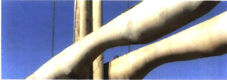
Figure 11: Fabric formwork creates architecturally interesting forms and can shape optimized beams (Credit: “Bespoke Reinforcement for New Concrete Structures” 2019)
