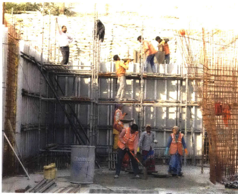
Figure 16: Many workers take part in a bucket brigade for pouring concrete (Credit: Ismail)
