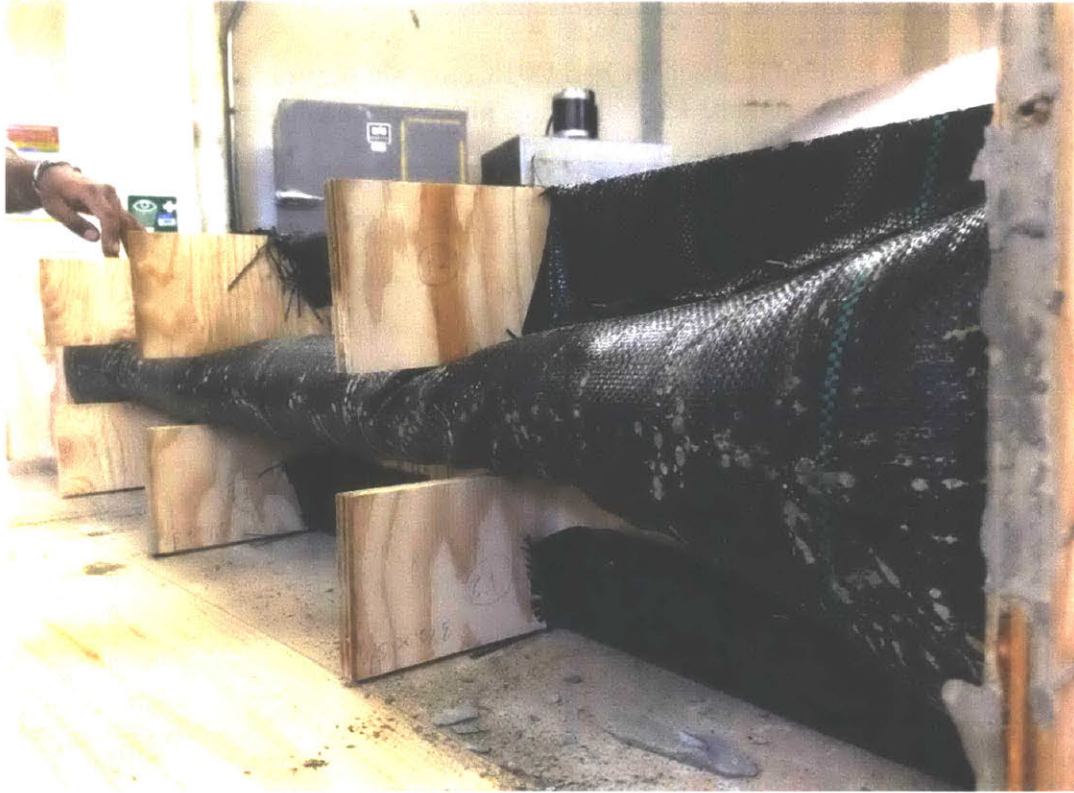
Bulging of the fabric formwork. Photo: Yan Liu.
