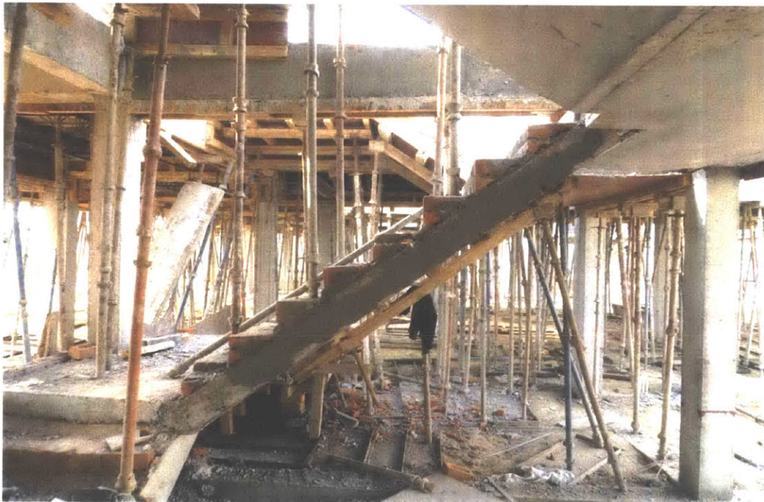
Staircases are cast concrete diagonal slabs with plastered-over bricks making up the stairs. Photo: Mohamed Ismail
