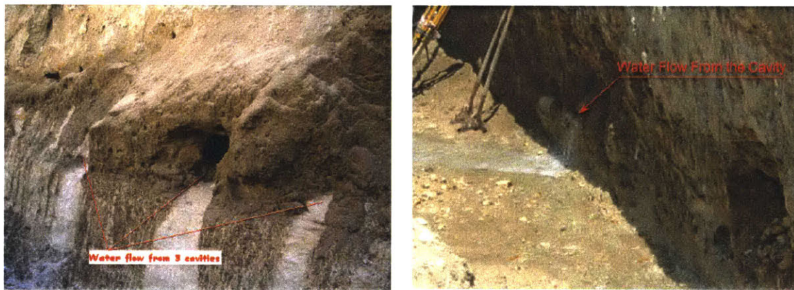
Figure 2-43: Groundwater flow from cavities [A.C.E.S., 2009].
