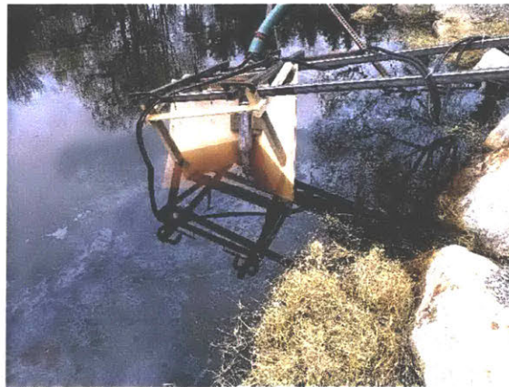
Figure 4-2: Photograph of the vee inlet in the water with hay ready to be pushed into it. Note the discoloration of the water in the bottom left corner. This was the hydraulic fluid that got into the pond when the motor was lowered into the water.
