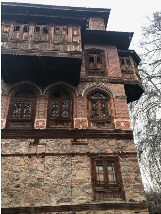
Figure 6.7 : Side Part of the Building from the kocha road leading to the Canal
