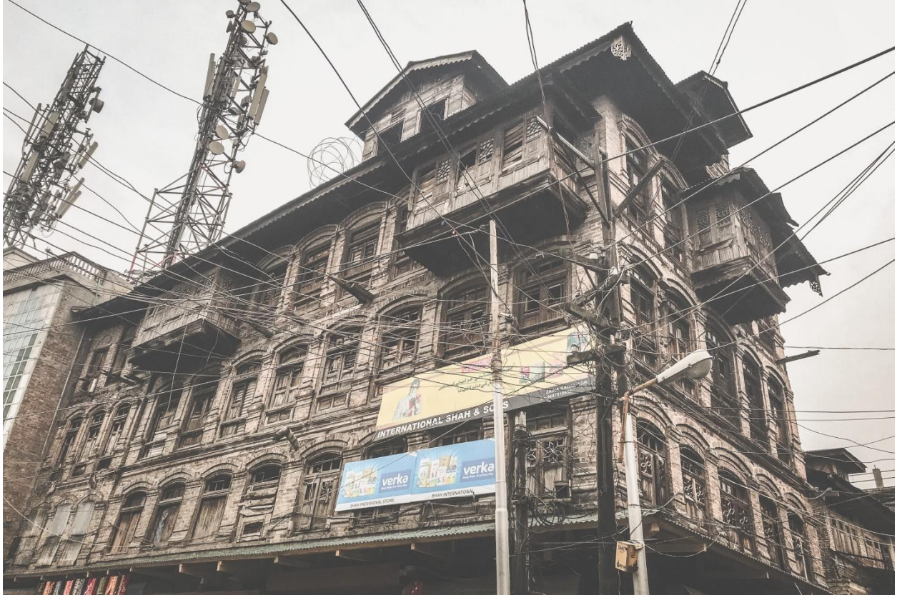
Figure 4.9: Building near Aali Kadal
