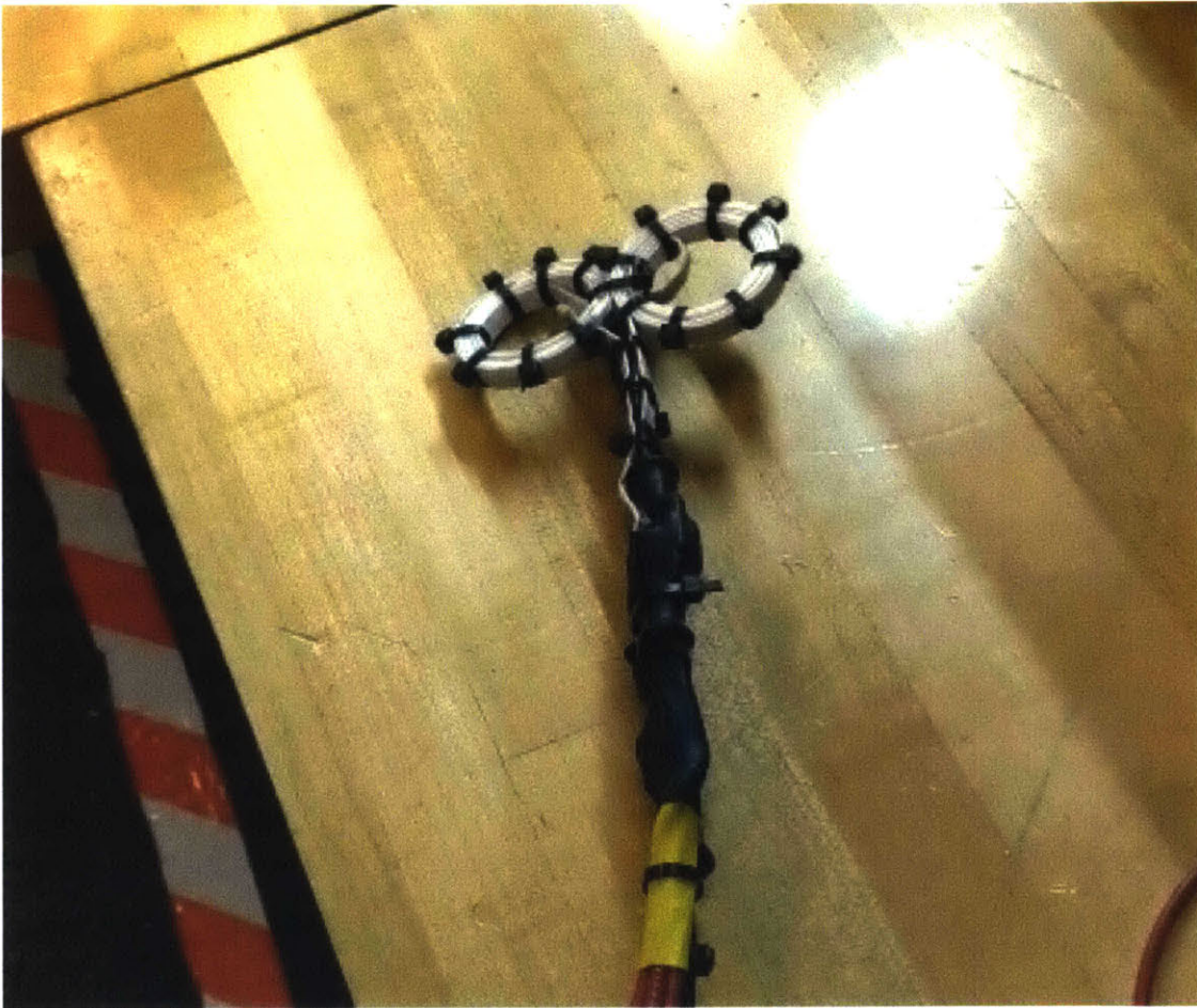
Figure 28: First of the 50mm coils in butterfly configuration.
